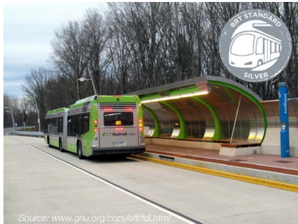
Figure 2-12: Cedar Street CTfastrak Station
