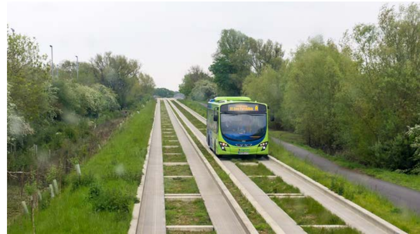
Figure 3-2: BRT in Cambridgeshire, UK has a path for walking and biking alongside the grassy BRT guideway
