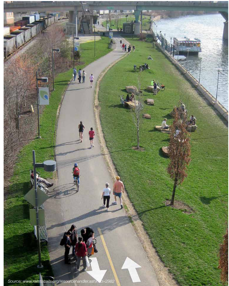
Figure 3-32: Rails-with-Trails often provide a safe travel alternative and reduce incentives to use the tracks as a shortcut.
