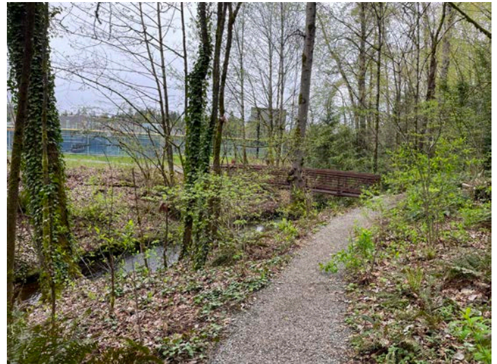
Existing bridge connecting to high school
