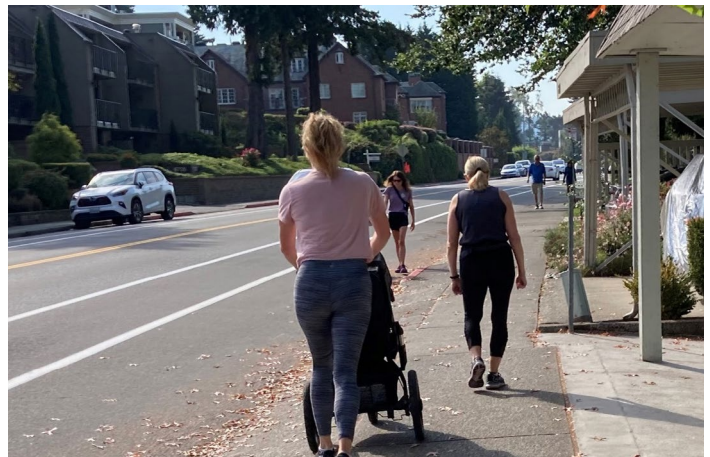
Narrow sidewalk at 5th Ave S
