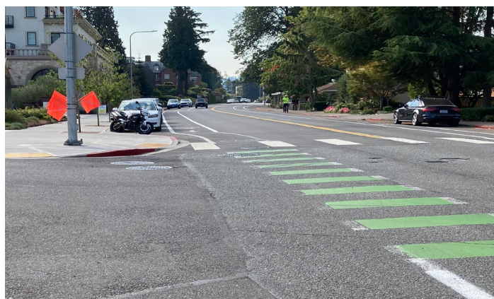
Northbound bike lane intersection at 10th Ave S is marked with green conflict markings for increased visibility of the bike lane for approaching drivers
