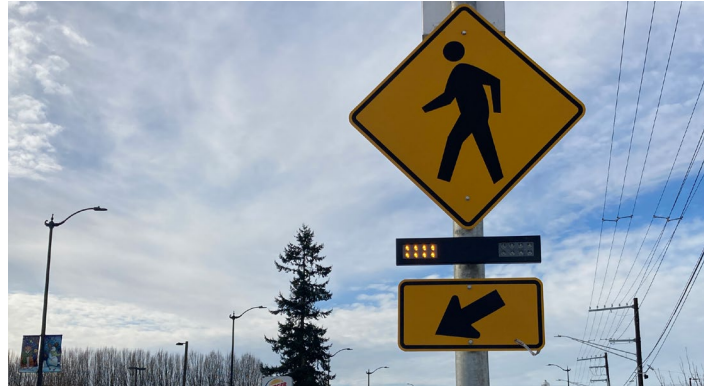
RRFB flashing lights increase crossing visibility
