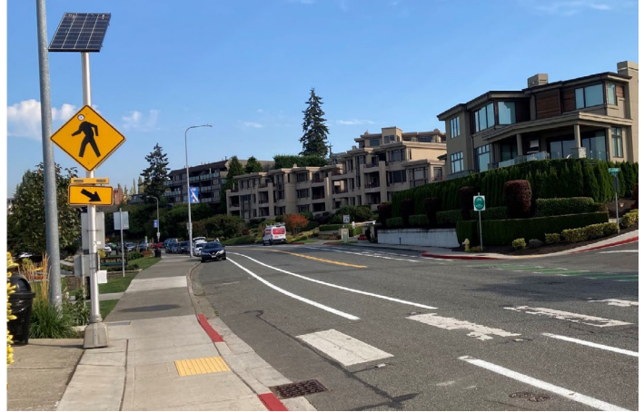
Sign mounted RRFB at 7th Ave S
