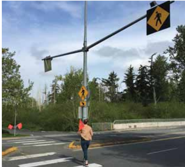
In Totem Lake, often there are long blocks between intersections with few safe pedestrian crossing opportunities. This mid block crossing on 116th Avenue NE facilitates a midblock street crossing with striping, signage, and a median refuge island.
