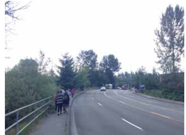
Totem Lake Boulevard is a major north-south arterial and bus corridor connecting destinations through the district. Sidewalks are very narrow and unpleasant to walk as there is no buffer between the sidewalk and the five vehicle lanes.
