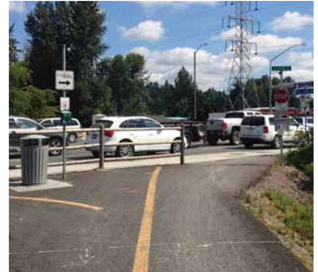
Presently the Cross Kirkland Corridor uses signage to direct trail users to an at-grade street crossing at NE 124th Street and 124th Ave NE. There are plans for a bicycle pedestrian bridge, also called the Totem Lake Connector, to continue over this intersection and maintain a trail experience.
