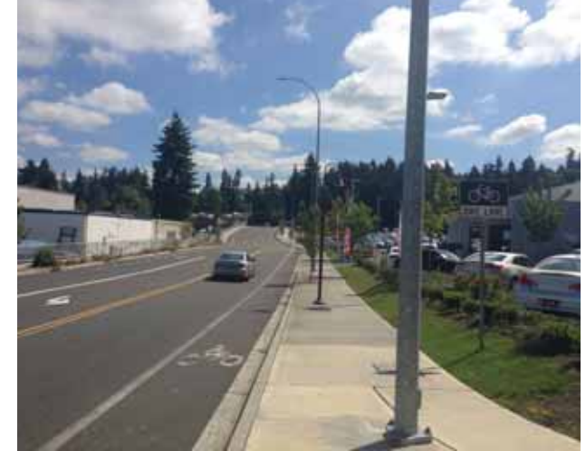
NE 120th St currently has three travel lanes and bike lanes, which represents LTS 3, comfortable for confident cyclists.
