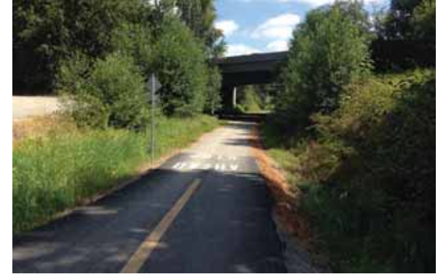
A future street connection is proposed in the ROW adjacent to the Cross Kirkland Corridor beneath Interstate 405.
