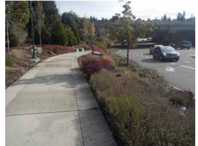
The newly constructed sidewalk on NE 116th has a diversity of plantings and trees, lighting, ample setback from the vehicle lanes, and wider walking space. Although 116th is a major arterial, these treatments make walking an enjoyable experience.
