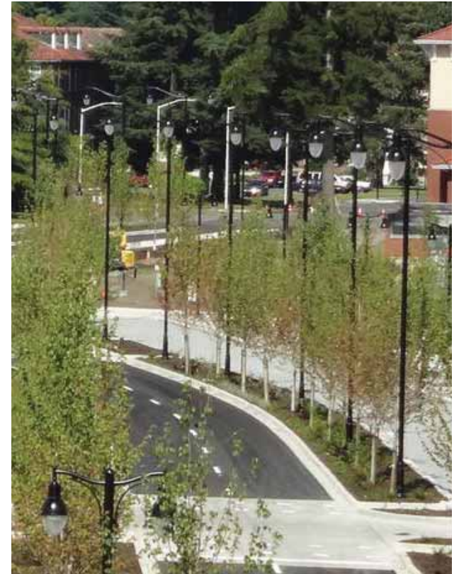
Consistent style and placement of light poles and trees distinguishes the character of this street, and acts as a breadcrumb wayfinding element. This strategy can be applied to the Circulator.
