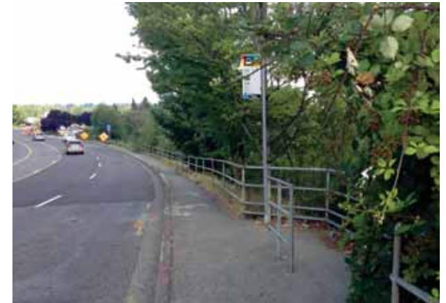
Most bus stops in Totem Lake are sign posts on the sidewalk and do not have amenities such as a shelter or seating area. This stop on Totem Lake Boulevard is an uninviting place to wait as the sidewalk is narrow and there is no place to sit. The City has received a TIB grant for 2019 to improve Totem Lake Boulevard with wider sidewalks, lighting, and other streetscape improvements.
