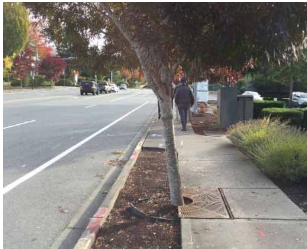
Street trees need at a minimum 4'6" for a full tree grate. Tree grates should not be a part of the clear walking zone.
