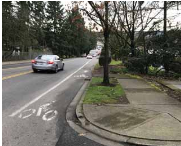
Some sidewalks abruptly end along property frontages, such as NE 120th St just east of Slater Ave.
