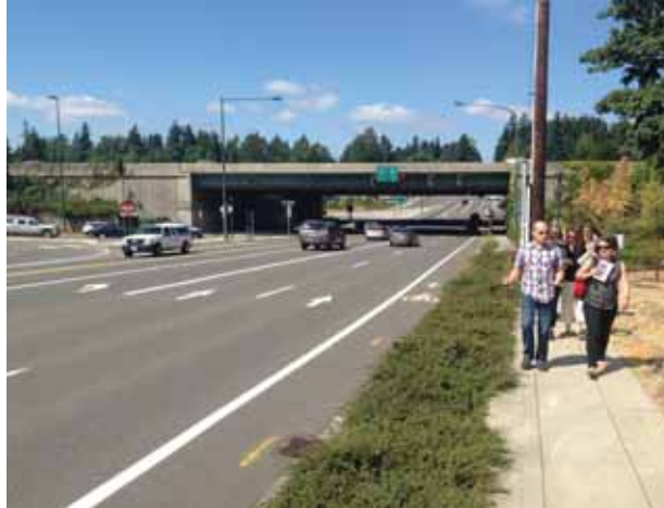
Comfortable walking and bicycling connections across Interstate 405 are critical to create cohesion across the Totem Lake district. NE 116th St, shown above, was recently improved with a widened sidewalk and planting buffer.
