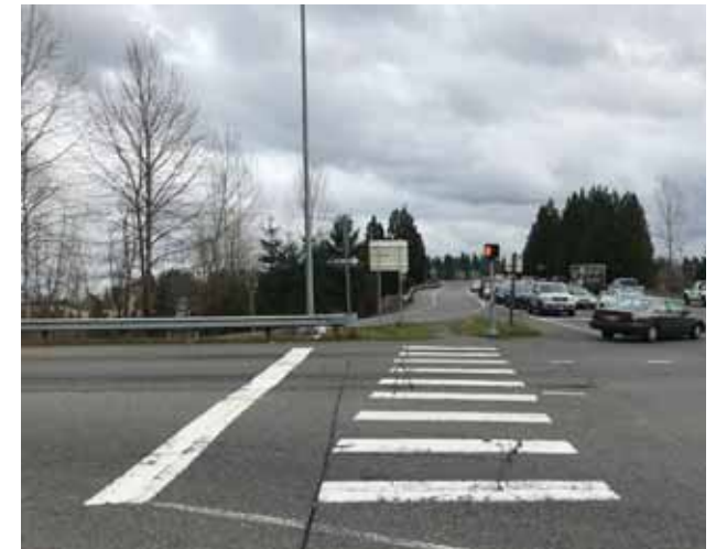
Though there is a crosswalk and pedestrian walk signal, there is no receiving curb ramp or sidewalk for people walking on NE 124th St and 116th Ave NE.
