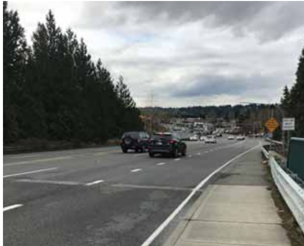
Some arterials in Totem Lake, such as NE 124th St, only have sidewalks on one side of the street. Note this particular sidewalk also abruptly ends in a shoulder.
