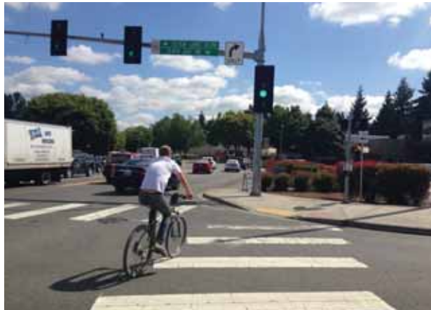
The current intersection of 124th Ave NE and NE 124th St does not have pavement markings to indicate bicycle crossing, a safe place to wait on the street, or directional curb ramps.
