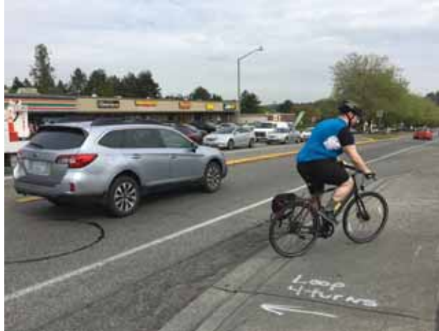
Recommended upgrades on the map are shown where an existing on street facility should be improved by adding separation between a bicycle lane and vehicle lanes. This encourages more people to ride who may not feel comfortable riding in a standard bike lane by reducing the route stress level to a 1 or 2. This image shows a cyclists exiting an existing bike lane on 124th Ave NE to ride on the sidewalk.
