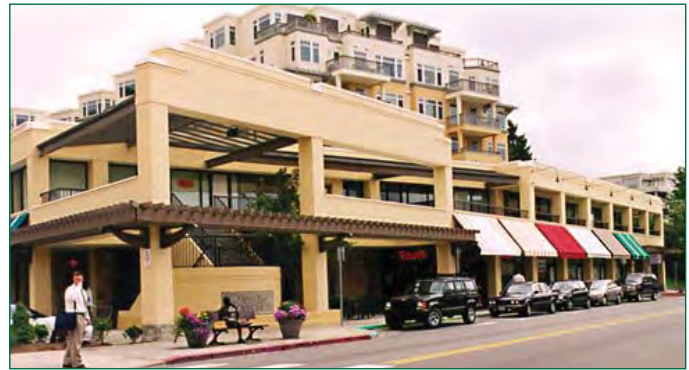
Horizontal modulation elements: canopy, brick banding, and window details.
