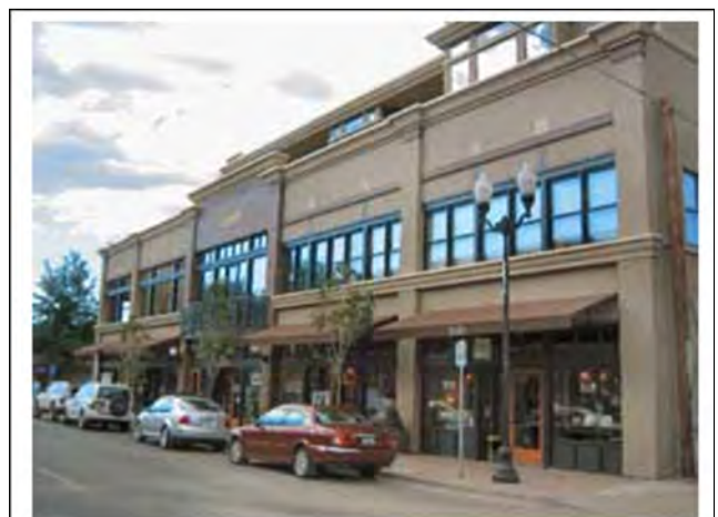
Figure 22. Note how these awnings have been integrated into the building's storefront spaces
