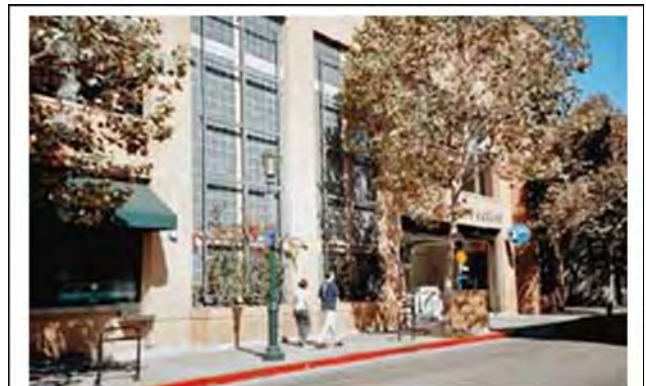
Figure 39. This parking garage includes streetfront retail space and landscaped trellises to mitigate visual impacts on the streetscape
