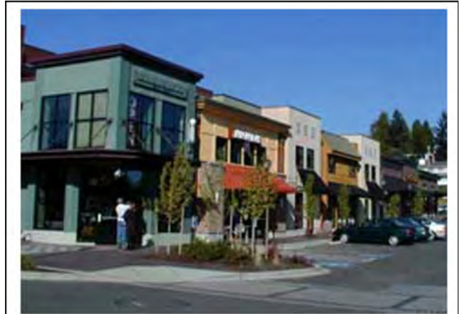
Figure 36. A variety of techniques should be used for multi-tenant retail buildings to emphasize individual storefronts
