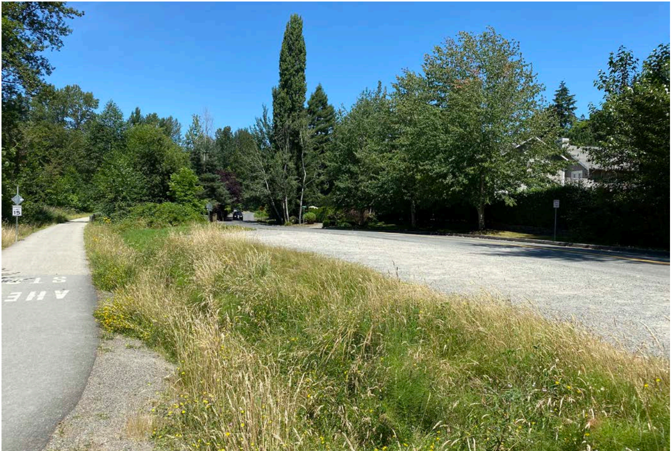
HLD 01 Sidewalk: 110th Avenue NE from Cross Kirkland Corridor to NE 97th Street
