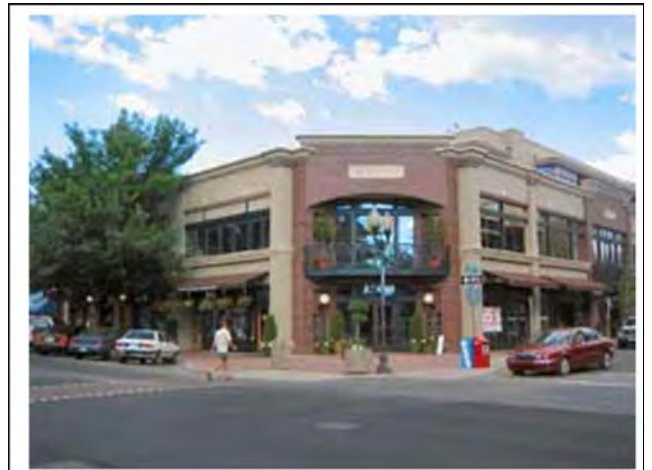
Figure 14. This building uses a cropped corner with entry and decorative roofline, building materials, and details to provide visual interest
