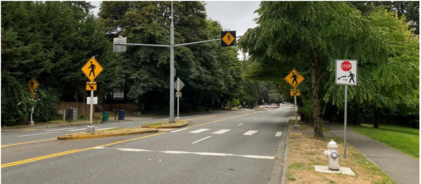
JN 02 Enhance crossing - Multi-lane Street: NE 124th Street at 102rd Avenue NE
