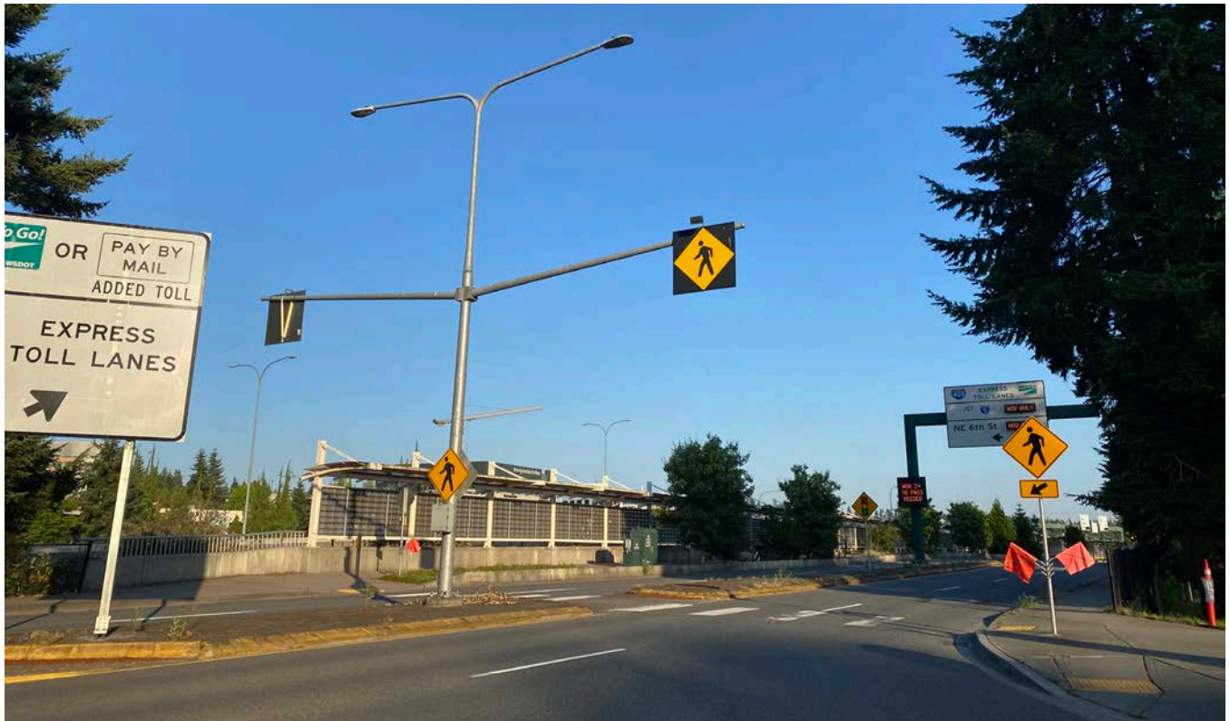
TL 01 Enhance crossing: 116th Avenue NE north of NE 128th Street
