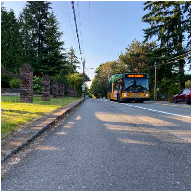
NRH 02 Sidewalk: 132nd Avenue NE from NE 110th Place to NE 97th Street
