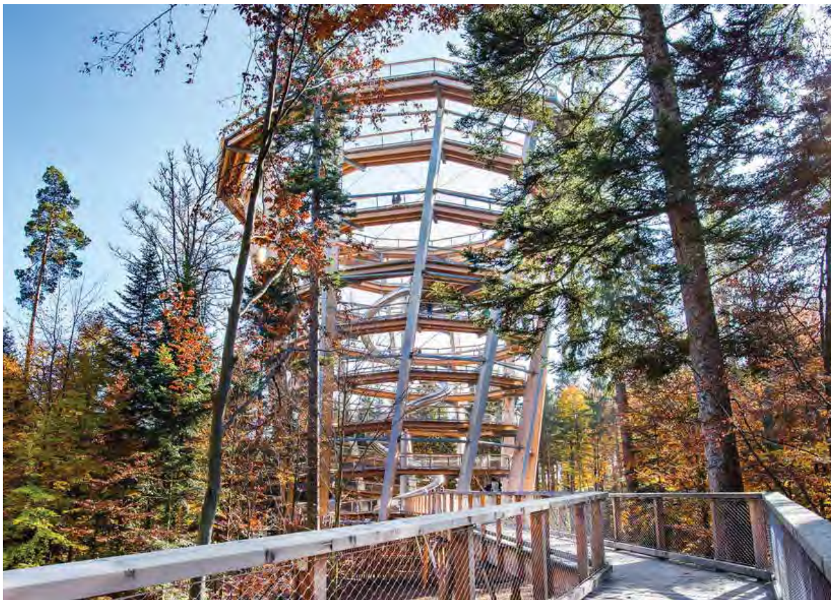
Figure – Example Spiral Lookout Tower in the Czech Republic
