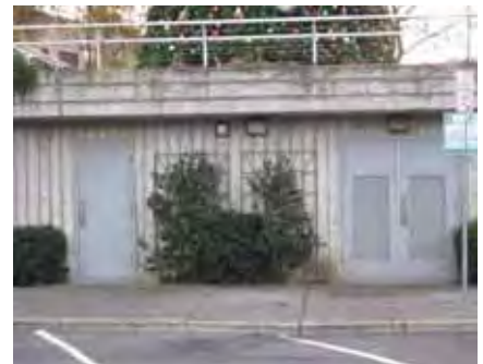
Lake Plaza Lift Station
