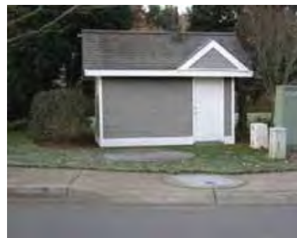
Yarrow Bay II Lift Station
