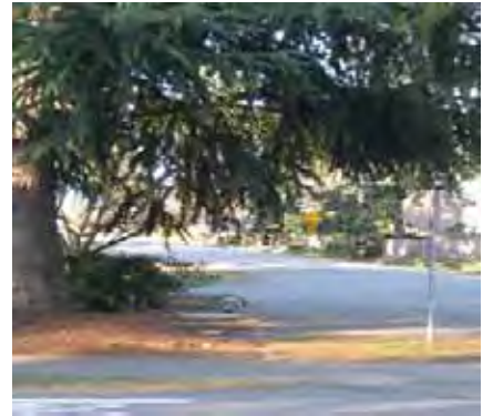
Trend Lift Station
