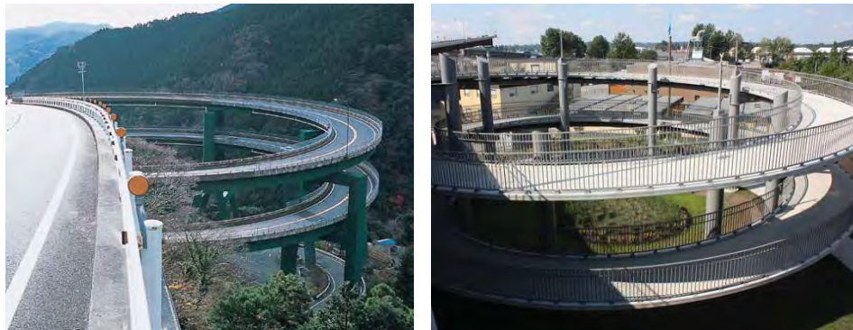
Figure – Spiral ramp examples for a roadway in Japan (L) and pedestrian ramp in British Columbia (R)
