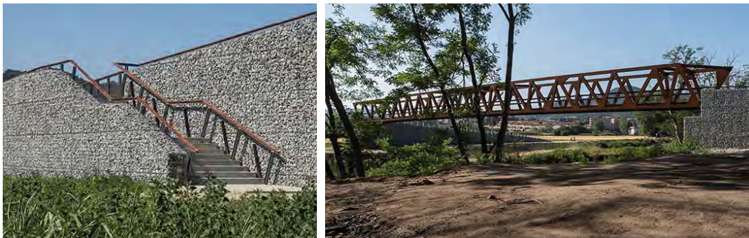
Figure – Wire-faced MSE walls artistically used on Montornes Pedestrian Bridge, Spain
