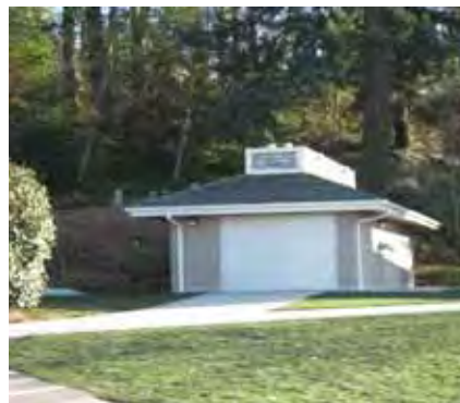
Waverly Park Lift Station
