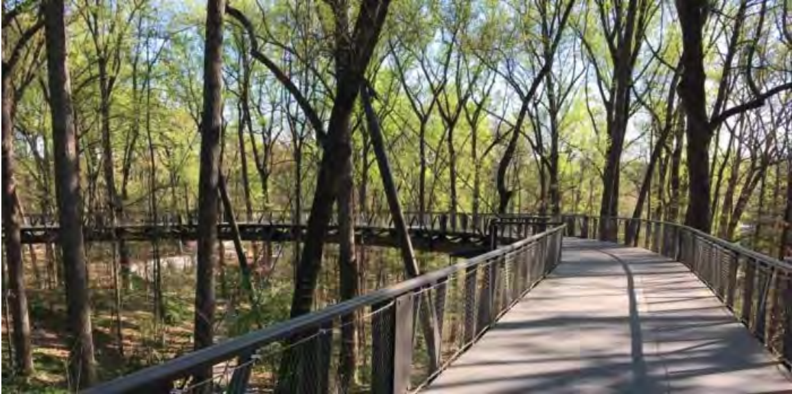
Figure – Atlanta Botanical Gardens Canopy Walk with 12-ft wide deck
