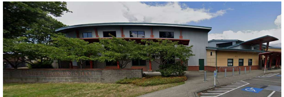
Lakeview Elementary School
