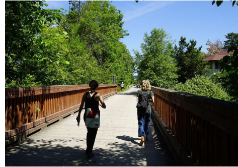
CKC Bridge over 68th Street
