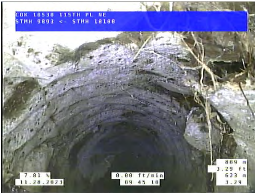
Site 1, Photo #2: 3.29 ft upstream of #10100
