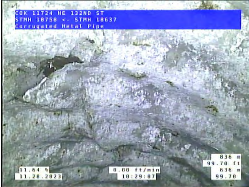
Site 2, Photo #7: 99.78 ft upstream of #10637
