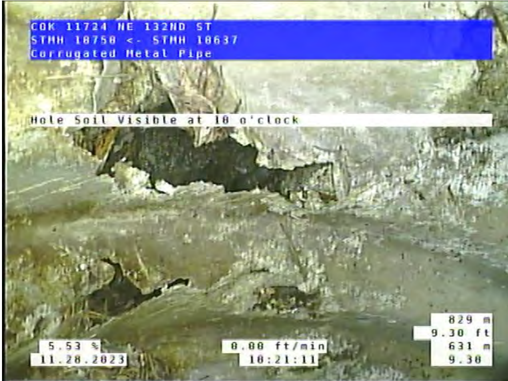
Site 2, Photo #3: 9.38 ft upstream of #10637
