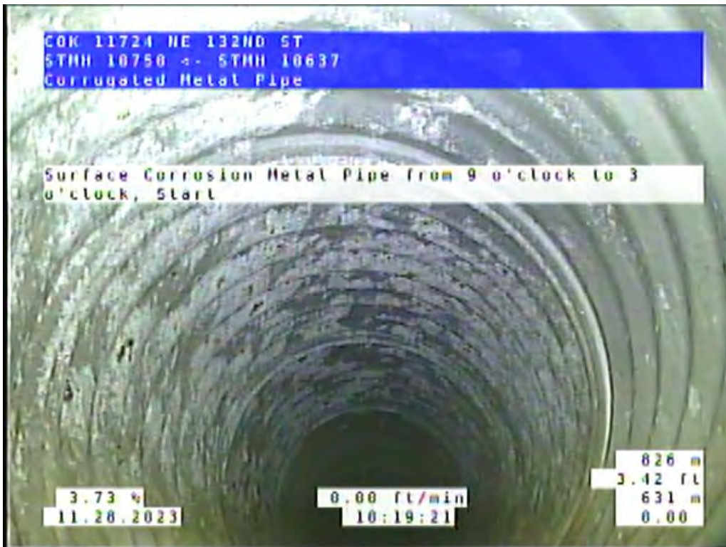
Site 2, Photo #1: 0.00 ft upstream of #10637
