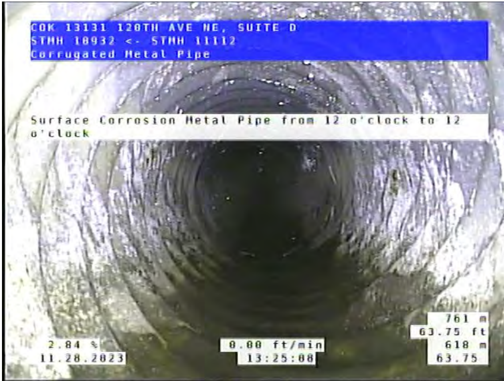
Site 4, Photo #2: 63.75 ft upstream of #11112
