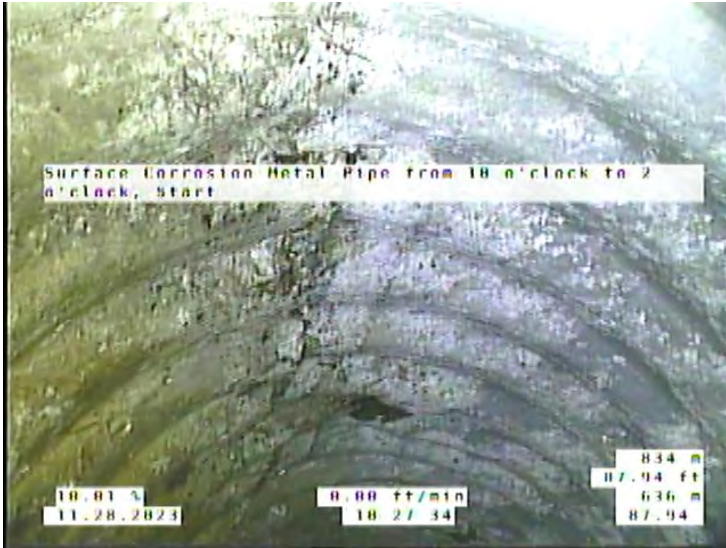
Site 2, Photo #6: 87.94 ft upstream of #10637
