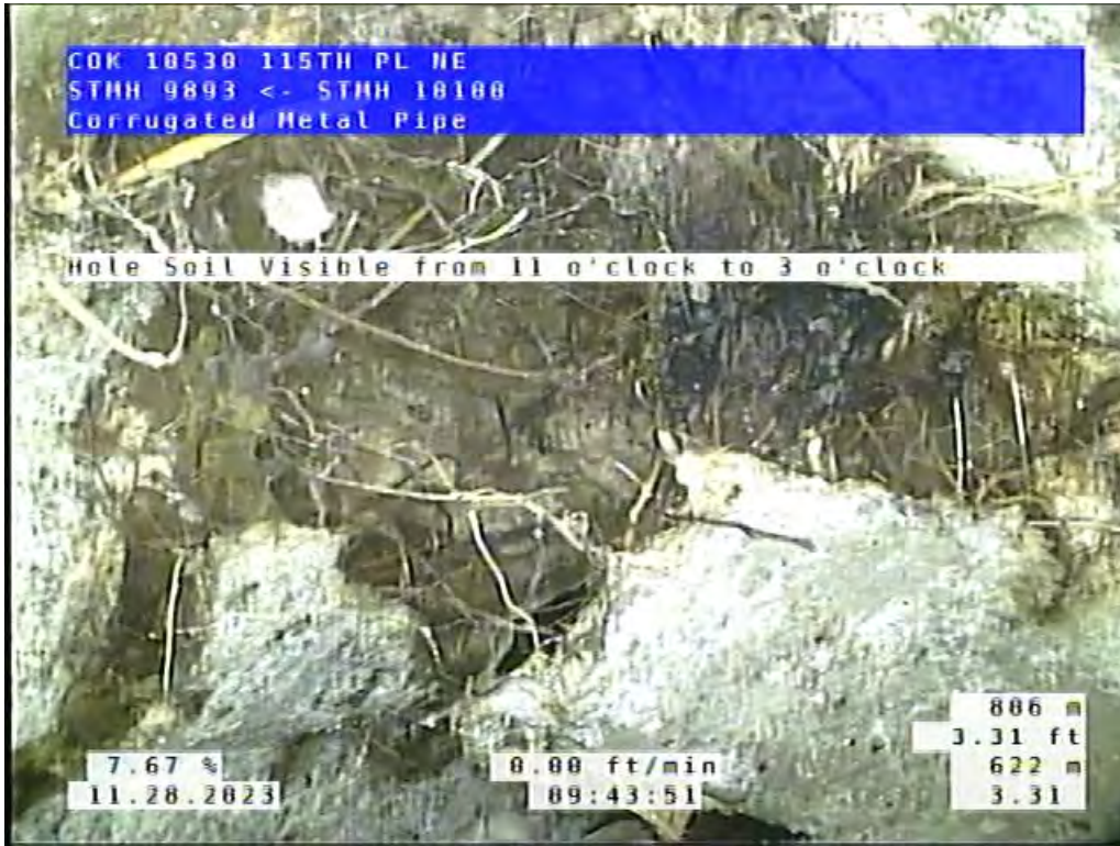
Site 1, Photo #3: 3.31 ft upstream of #10100
