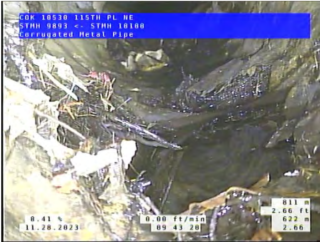
Site 1, Photo #1: 2.66 ft upstream of #10100
