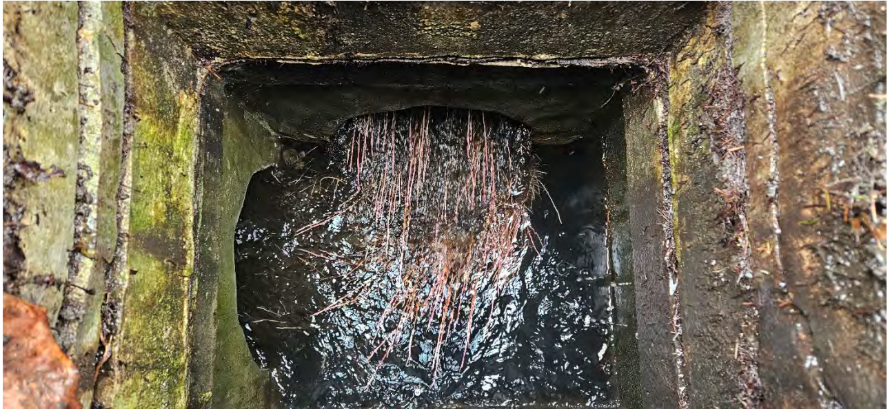
Site 2, CB#10750 –Type 1 catch basin (direction north at top image)
