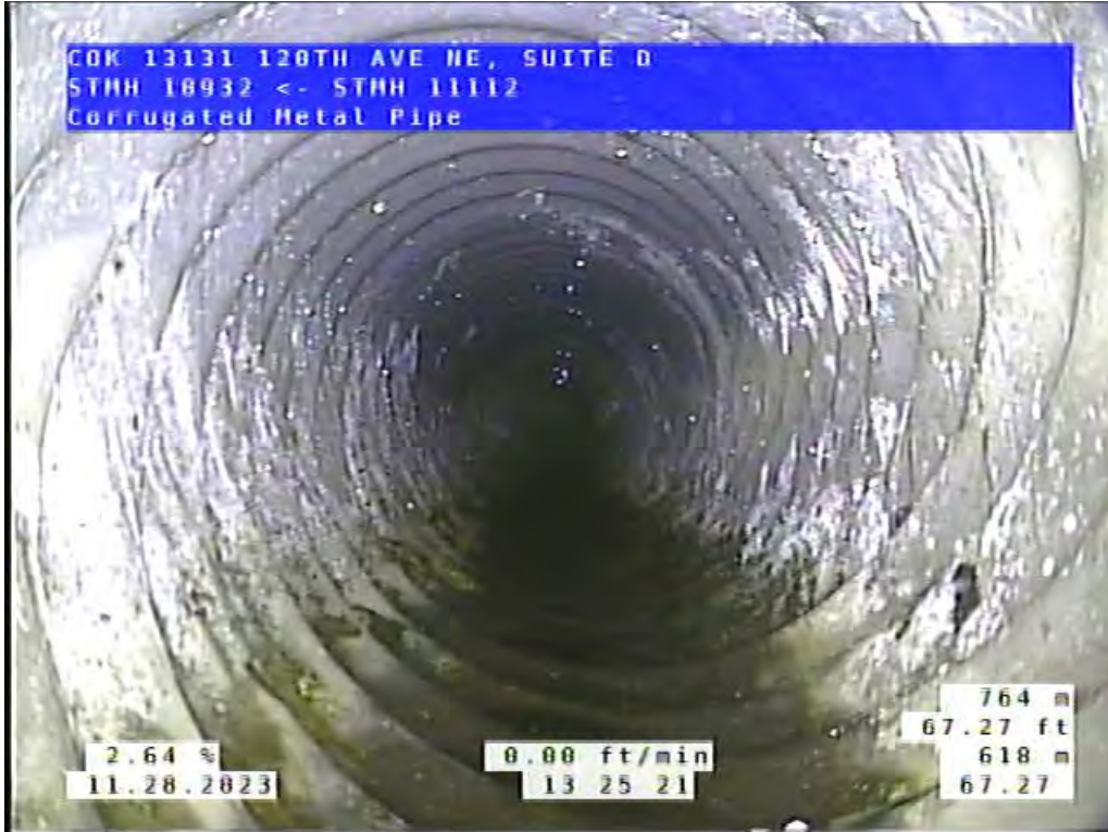
Site 4, Photo #3: 67.27 ft upstream of #11112
