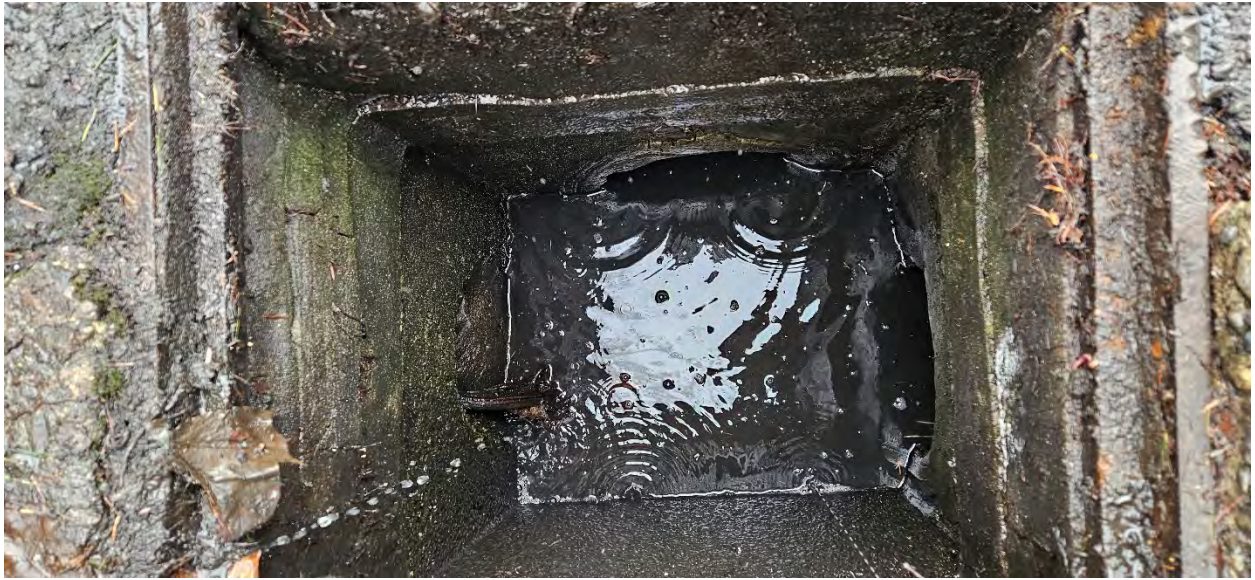
Site 3, CB#10849 –Type 1 catch basin (direction north at top image)
