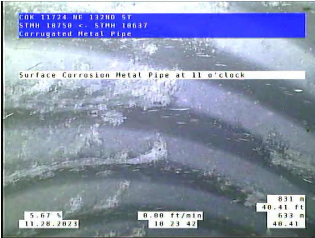
Site 2, Photo #4: 48.41 ft upstream of #10637
