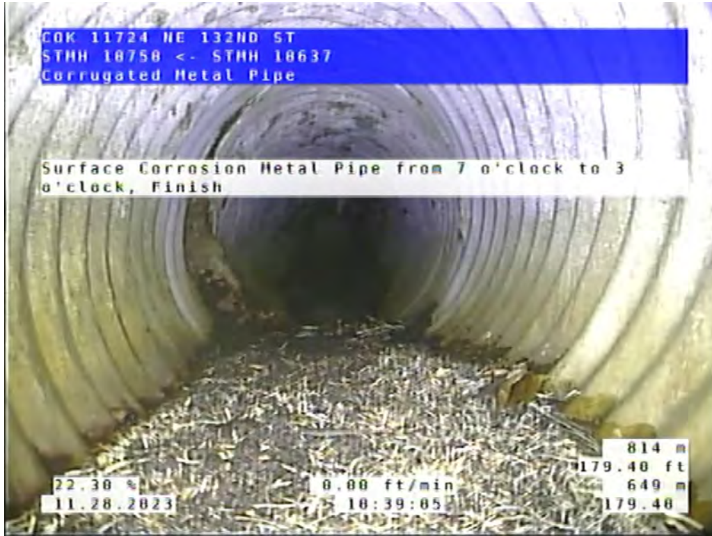
Site 2, Photo #8: 179.40 ft upstream of #10637
