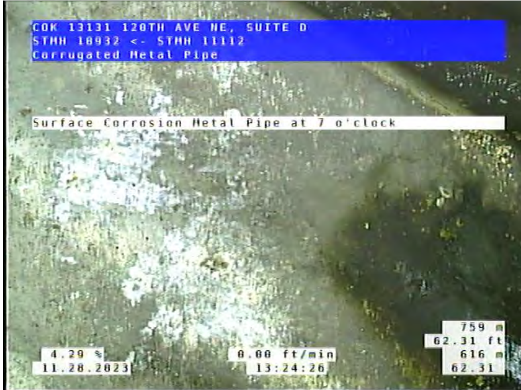
Site 4, Photo #1: 62.31 ft upstream of #11112
