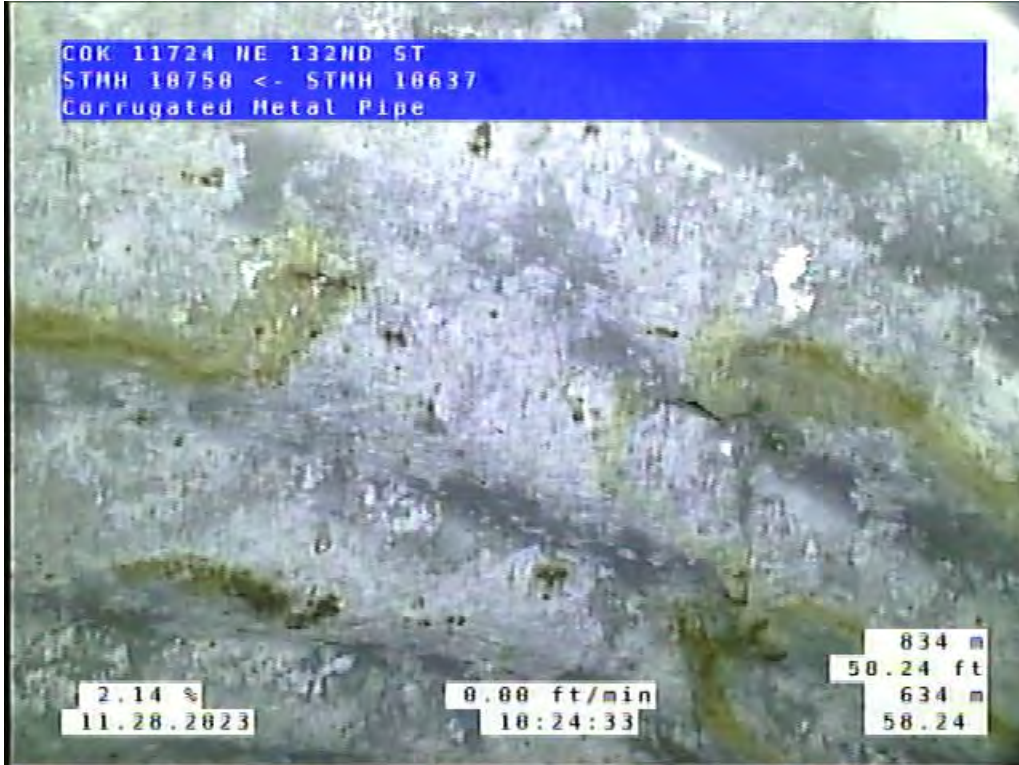
Site 2, Photo #5: 58.24 ft upstream of #10637
