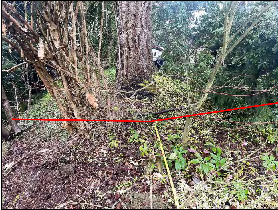
Photograph 1. The base of tree G with the approximate location of layback excavation indicated by the red line.
