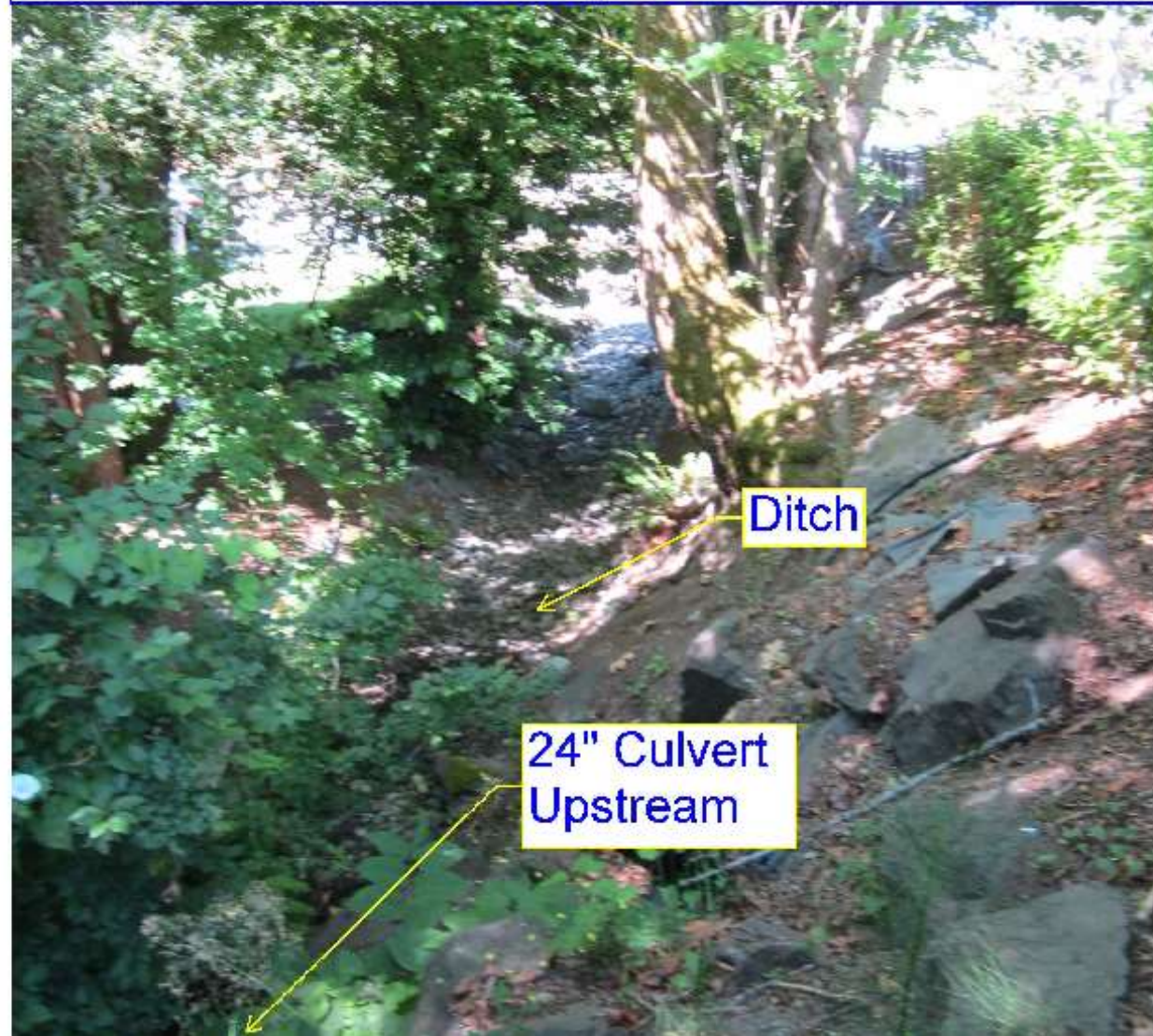
PHOTO #3, TDA2 - 18" Culvert Outfall Looking West
