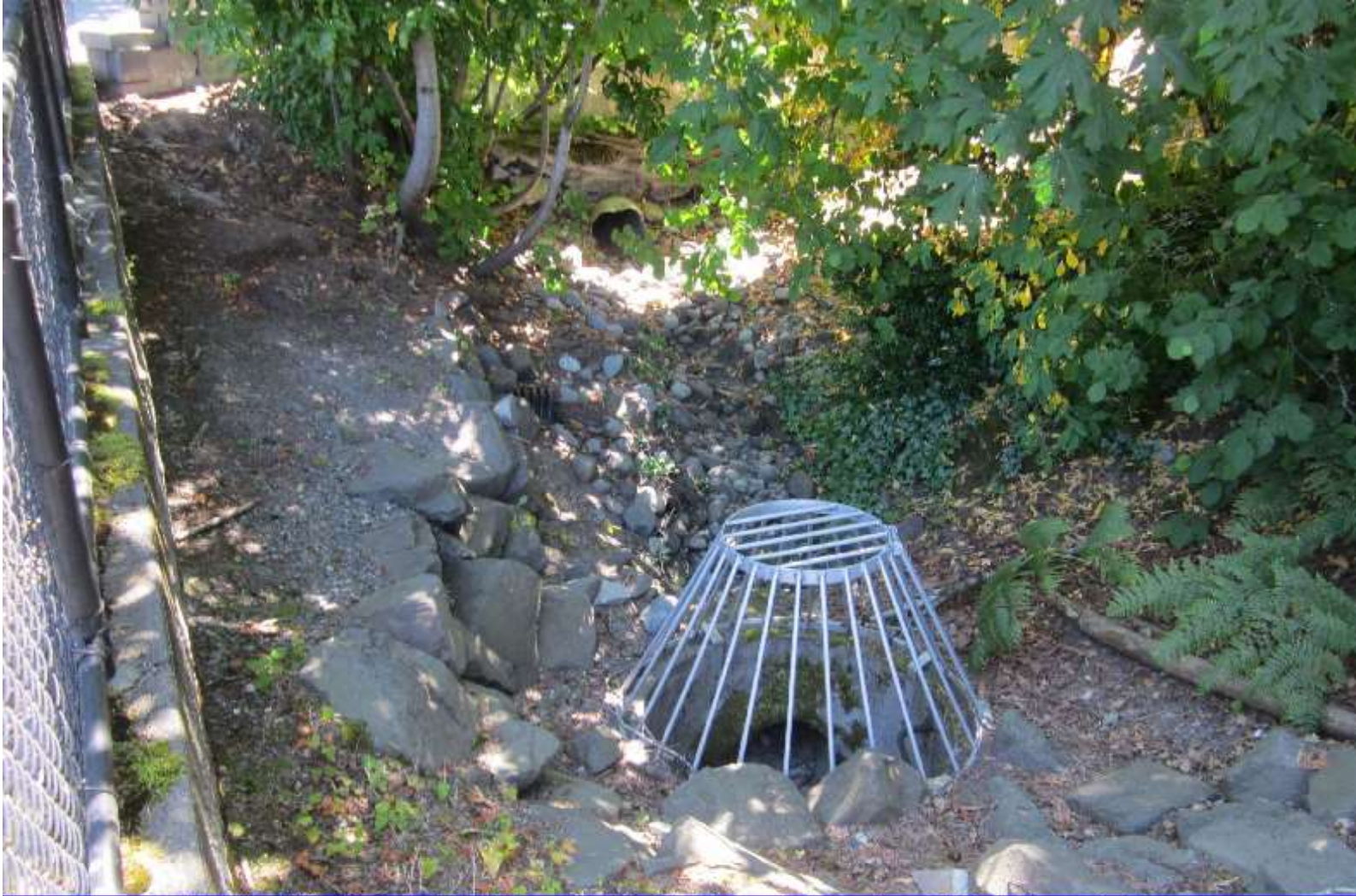
PHOTO #4, TDA2 - 24" Culvert Inlet at Kirkland Ave. Looking Upstream/Southeast
