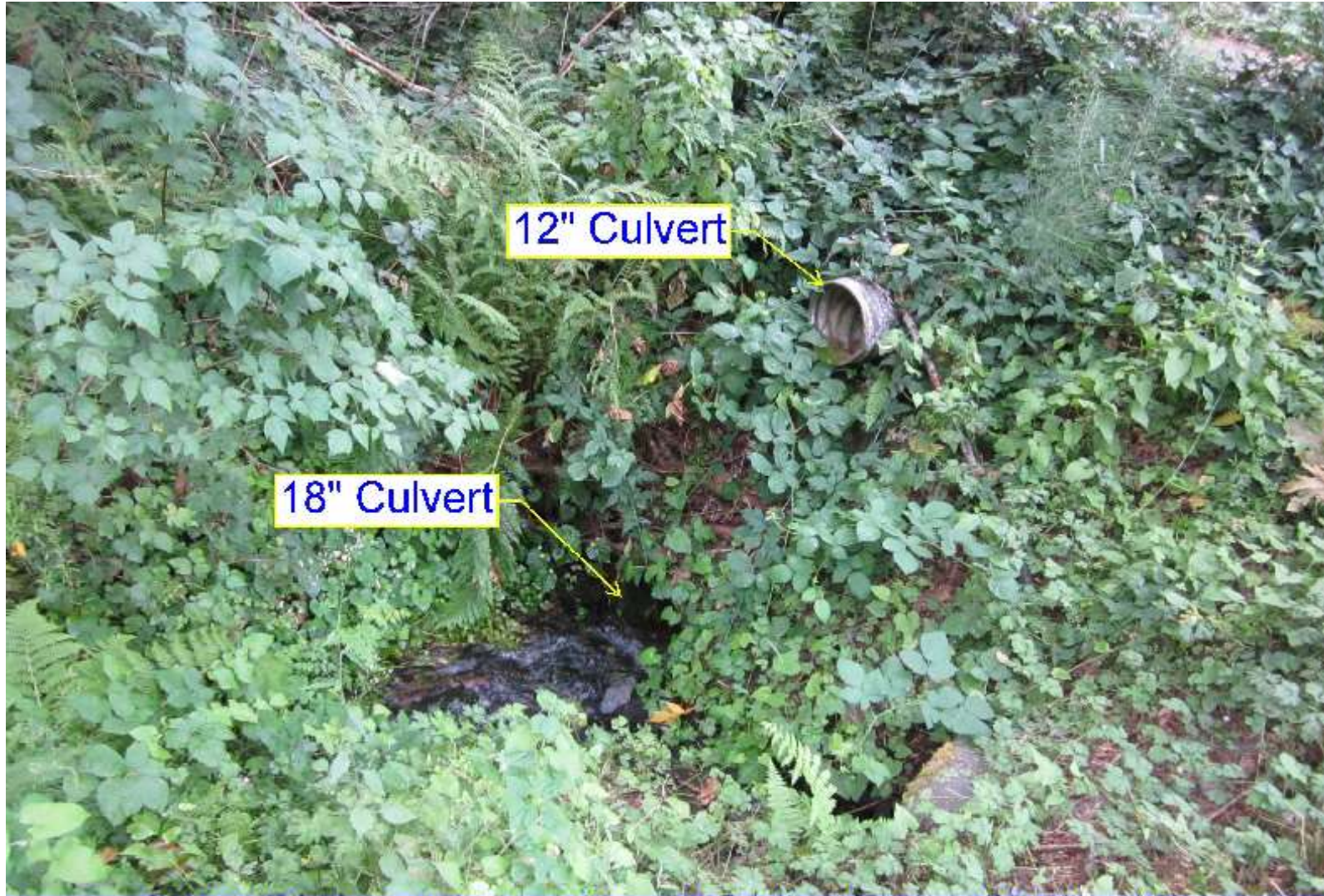
PHOTO #2, TDA1 - 18" and 12" Culverts at Slater St. Looking West
