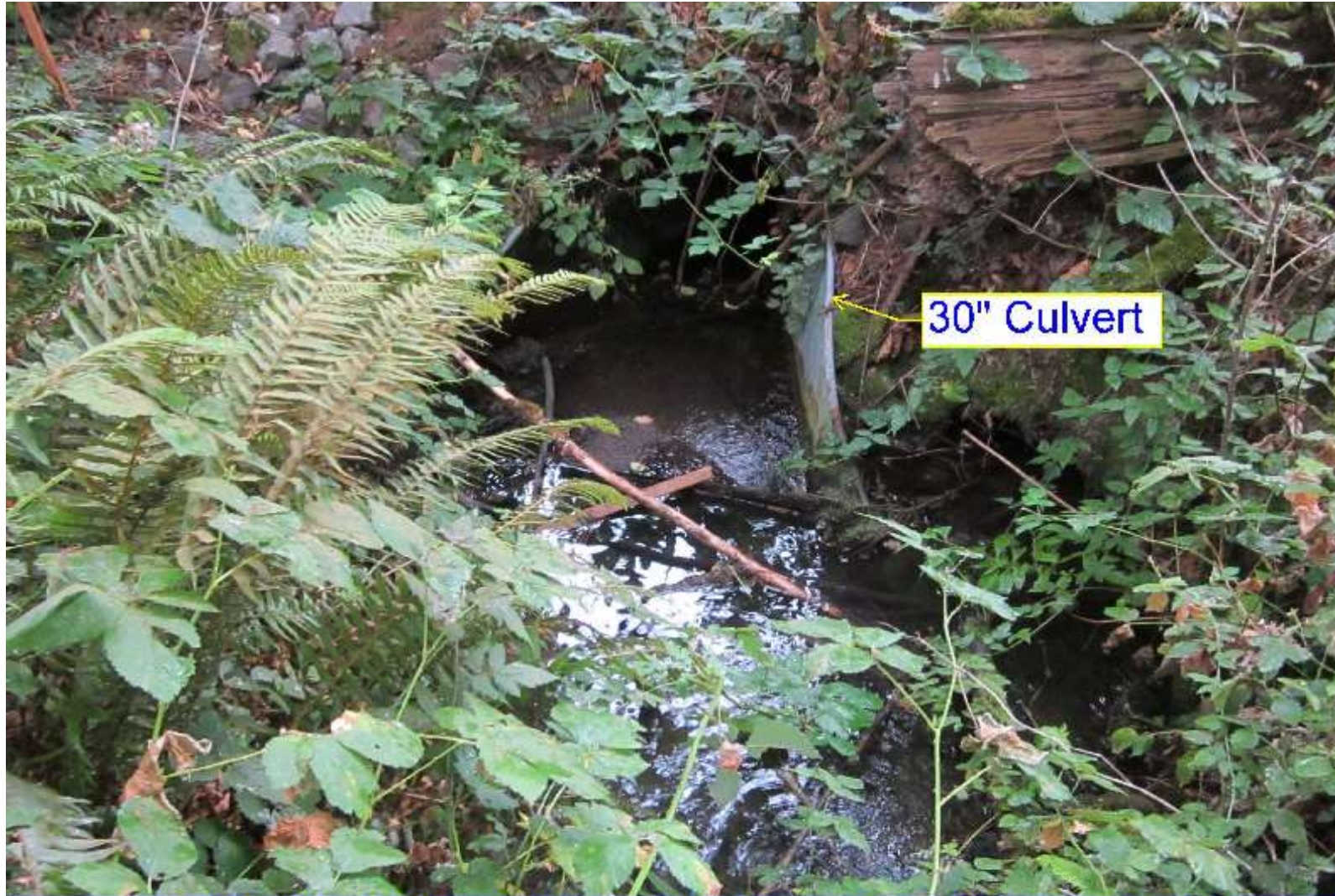
PHOTO #1, TDA1 - 30 Inch Culvert Inlet at Alexander Ave Looking Northwest
