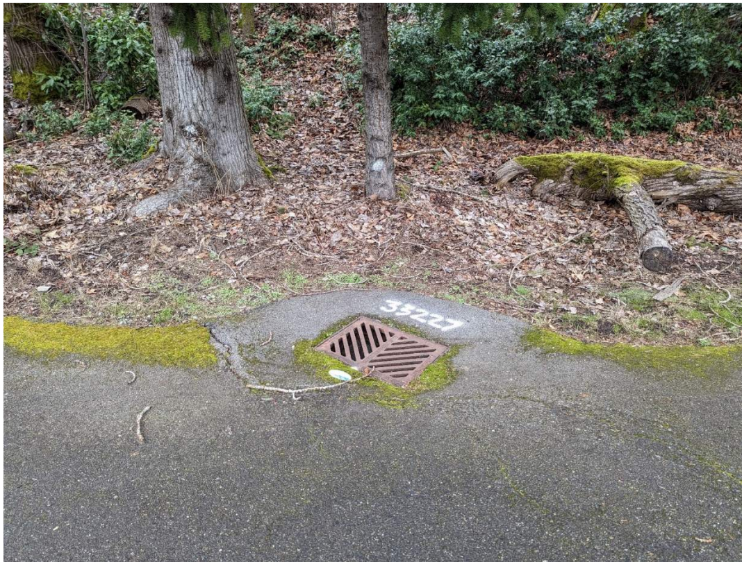
Photo 11. Catch basin on pedestrian path south of 85th.
