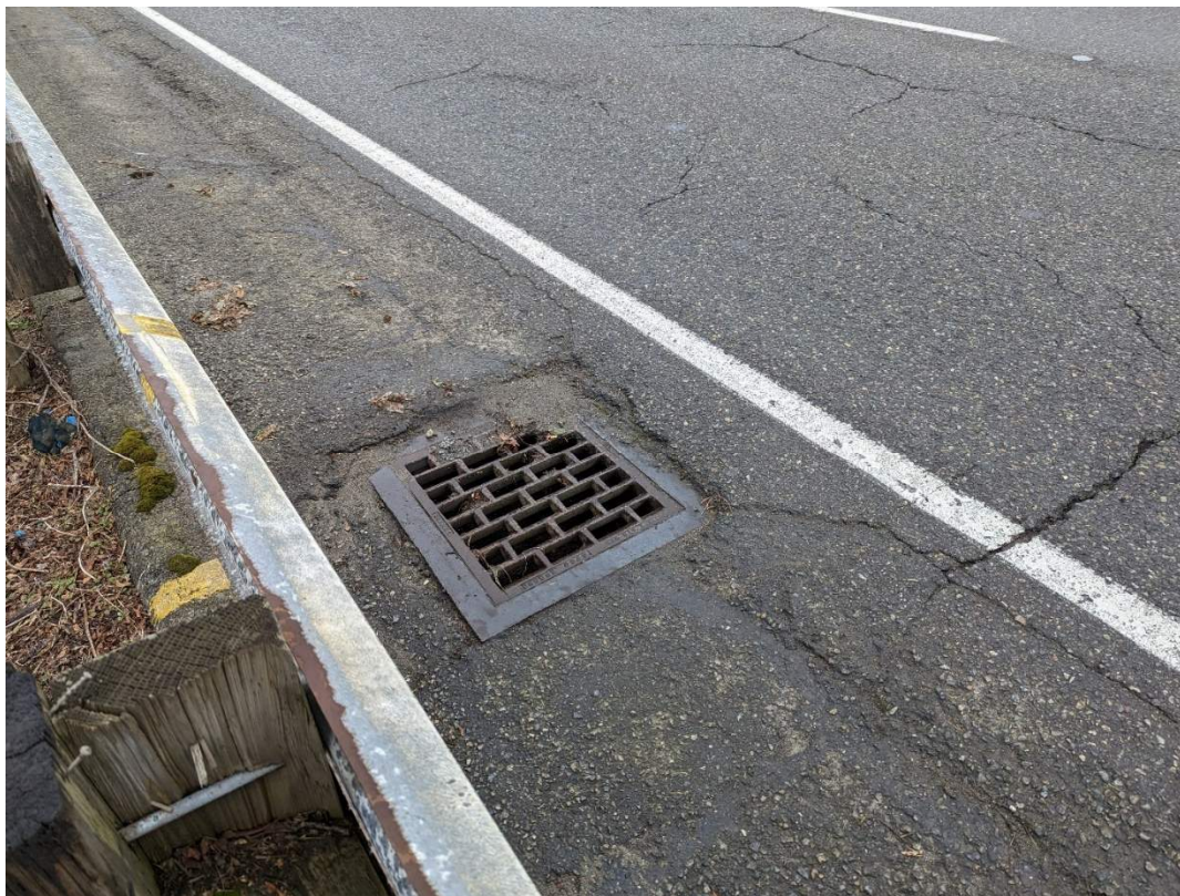
Photo 8. Discharge point on south side, just west of the bridge.
