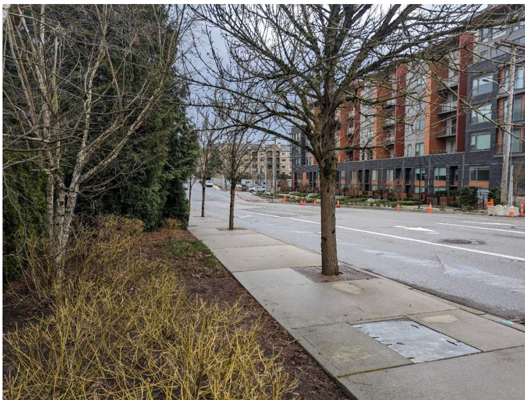
Photo 14. 6th Street looking south. Shown on the middle right side of the picture in the middle lane is the catch basin where the downstream discharge routes combine.
