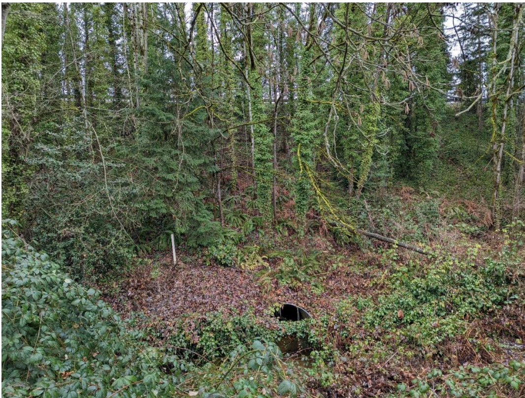
Photo 10. Outfall location south of 85th.
