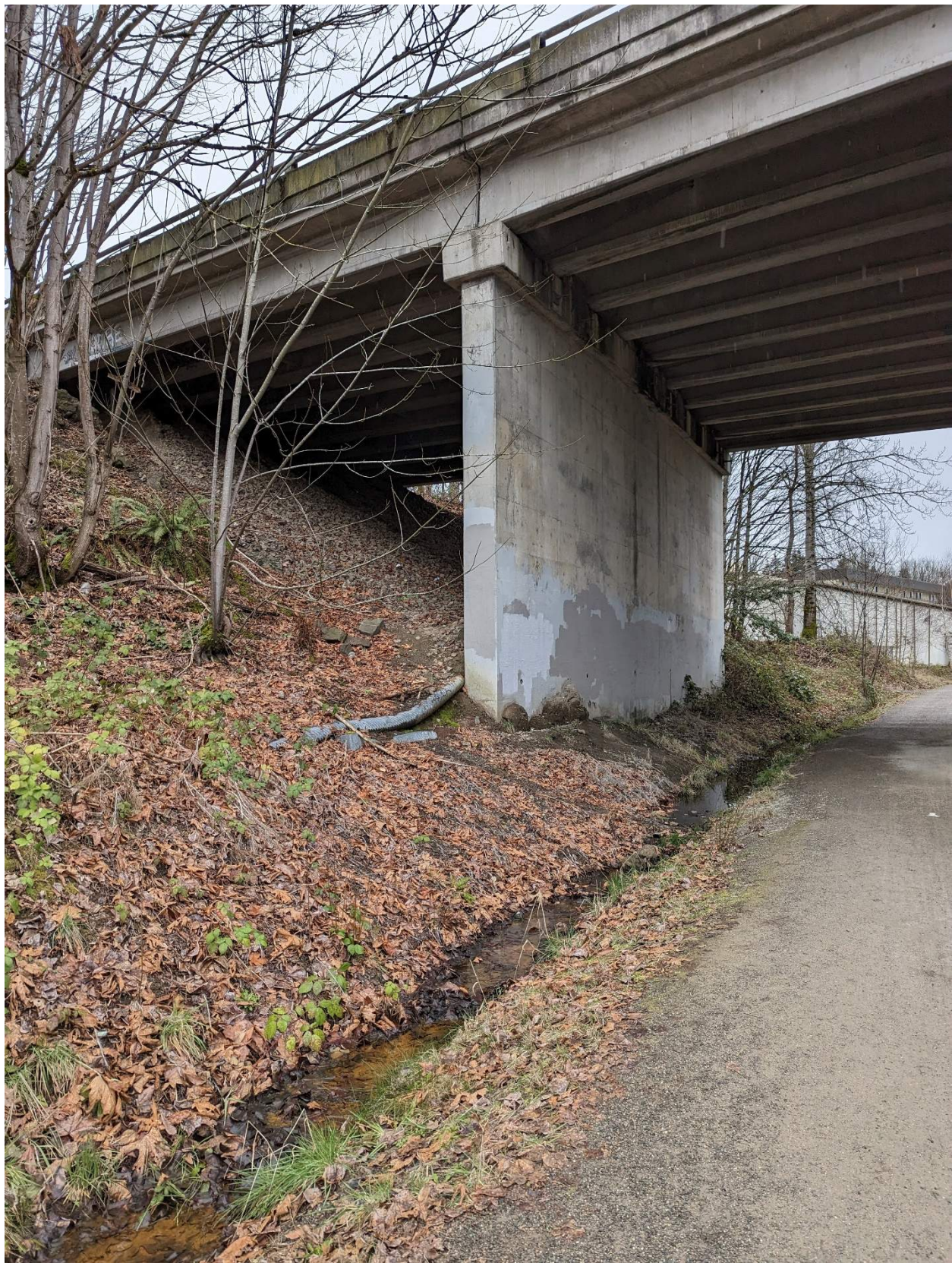
Photo 4. Drainage ditch under bridge on CKC near east end of project. Leaves TDA limits and flows north.
