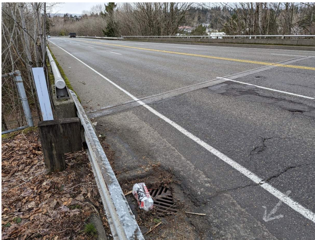
Photo 7. Catch basin on south side of road just east of the bridge.
