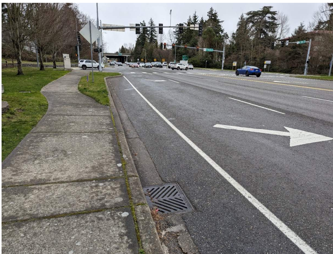
Photo 6. Discharge location near intersection of 85th and 114th.
