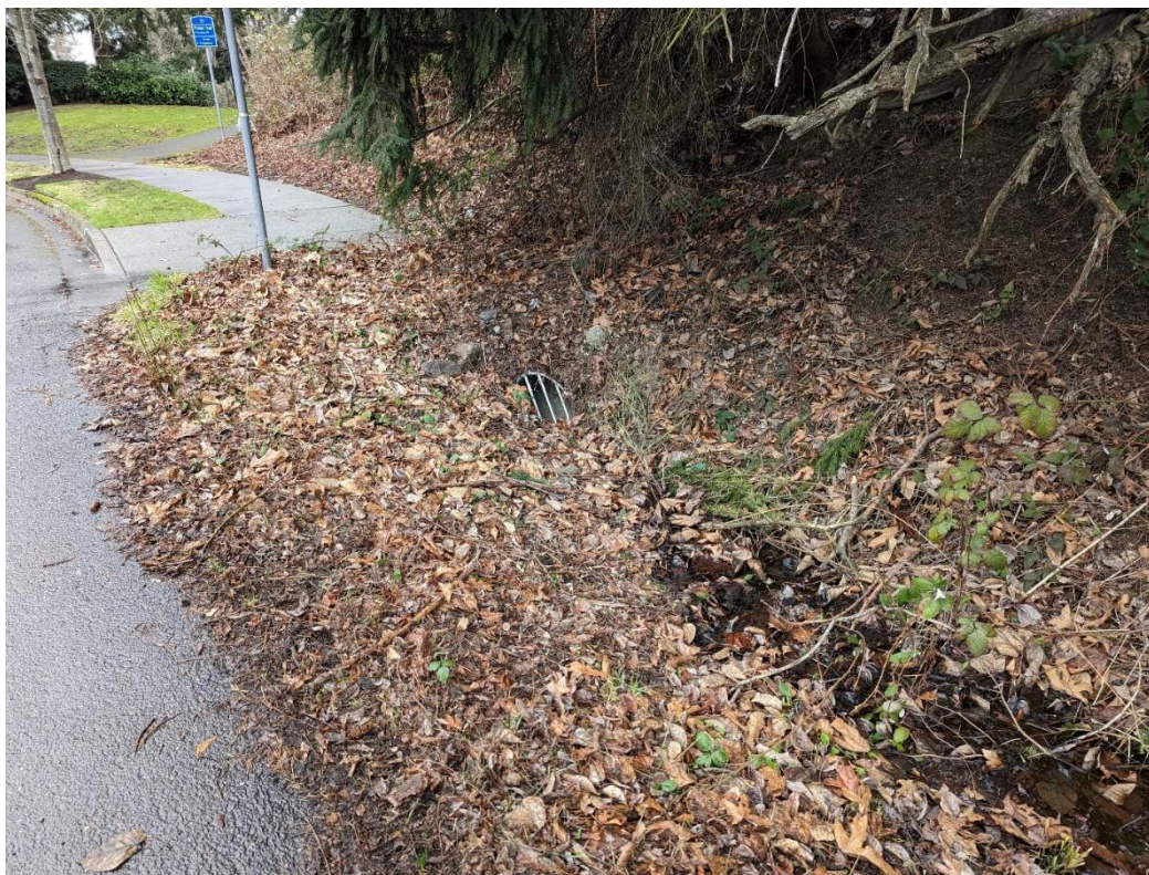
Photo 13. Ditch enters tightline conveyance system south of 85th.
