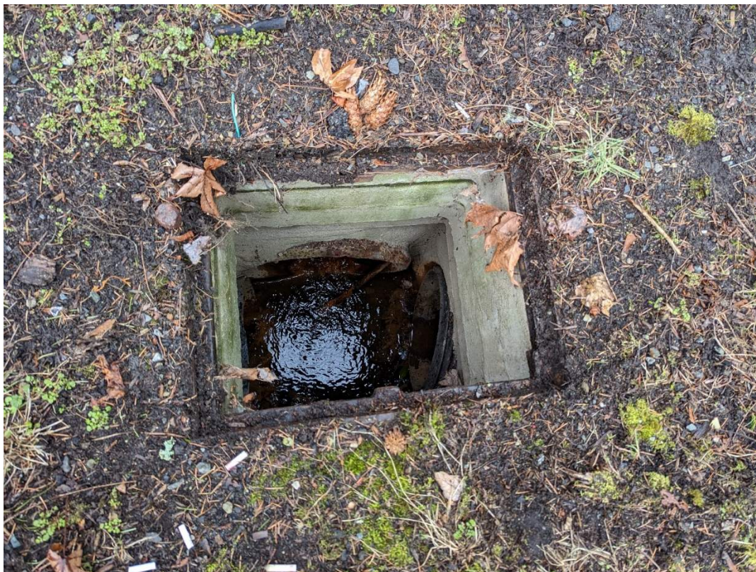
Photo 12. Catch basin along pedestrian path.
