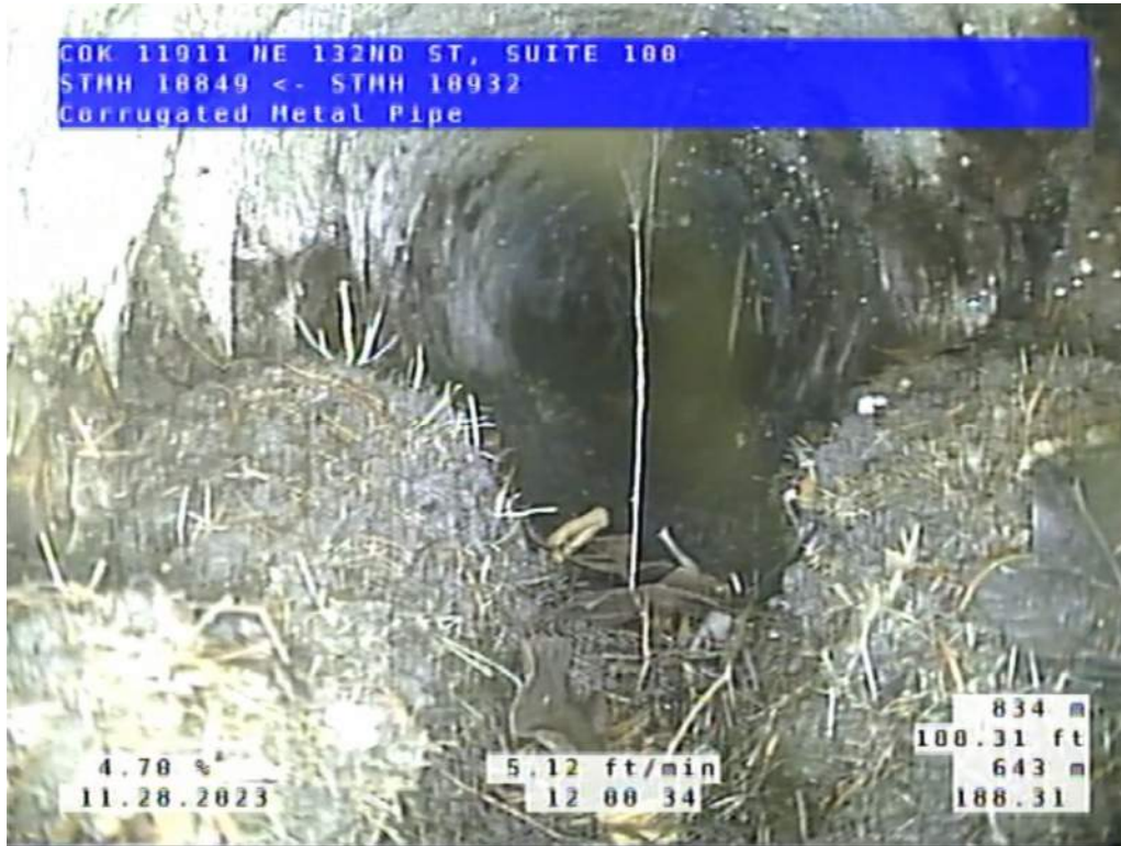
Site 3, Photo #4: 188.31 ft downstream of #10932
