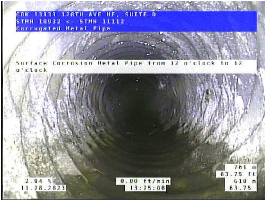
Site 4, Photo #2: 63.75 ft upstream of #11112
