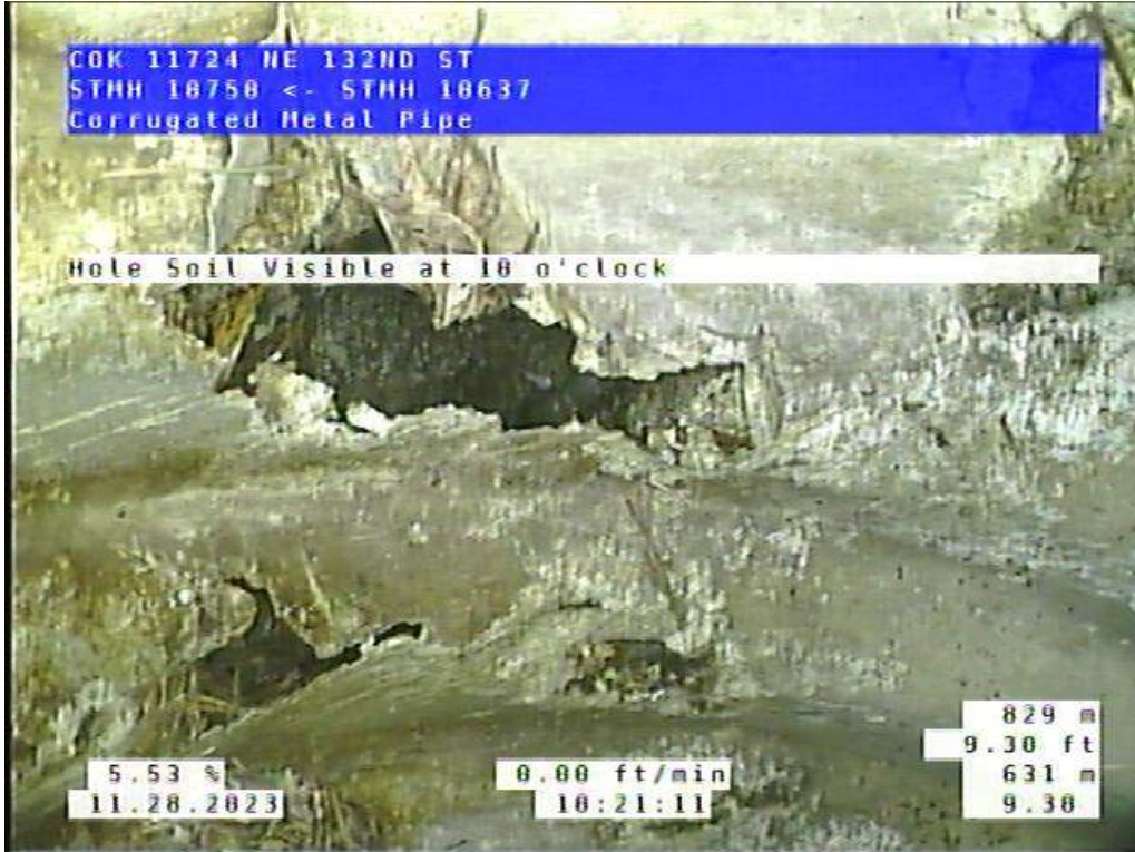
Site 2, Photo #3: 9.38 ft upstream of #10637
