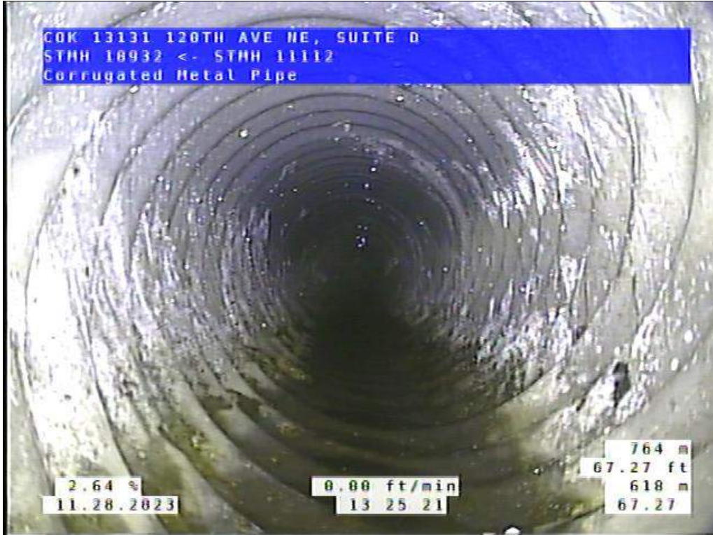
Site 4, Photo #3: 67.27 ft upstream of #11112
