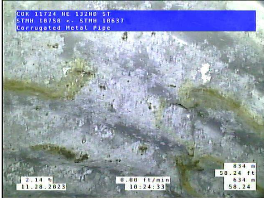
Site 2, Photo #5: 58.24 ft upstream of #10637
