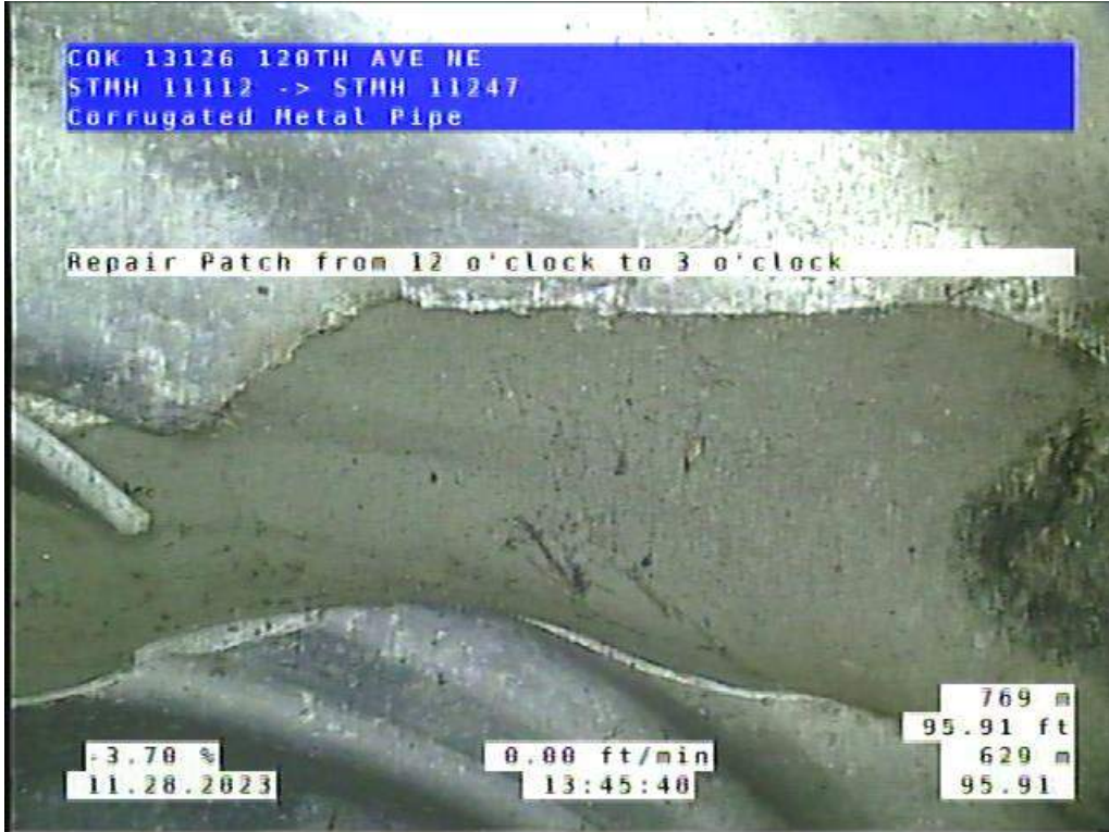
Site 5, Photo #6: 95.91 ft downstream of #11112
