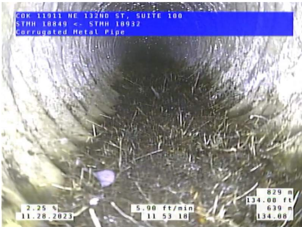
Site 3, Photo #3: 134.08 ft downstream of #10932
