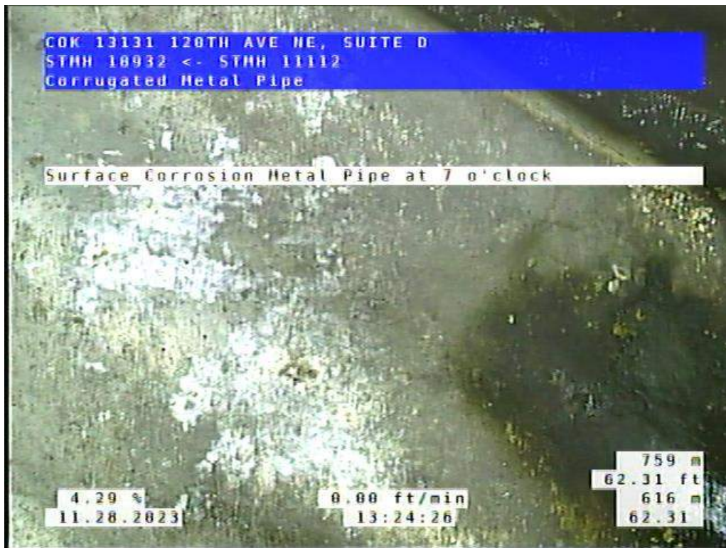
Site 4, Photo #1: 62.31 ft upstream of #11112
