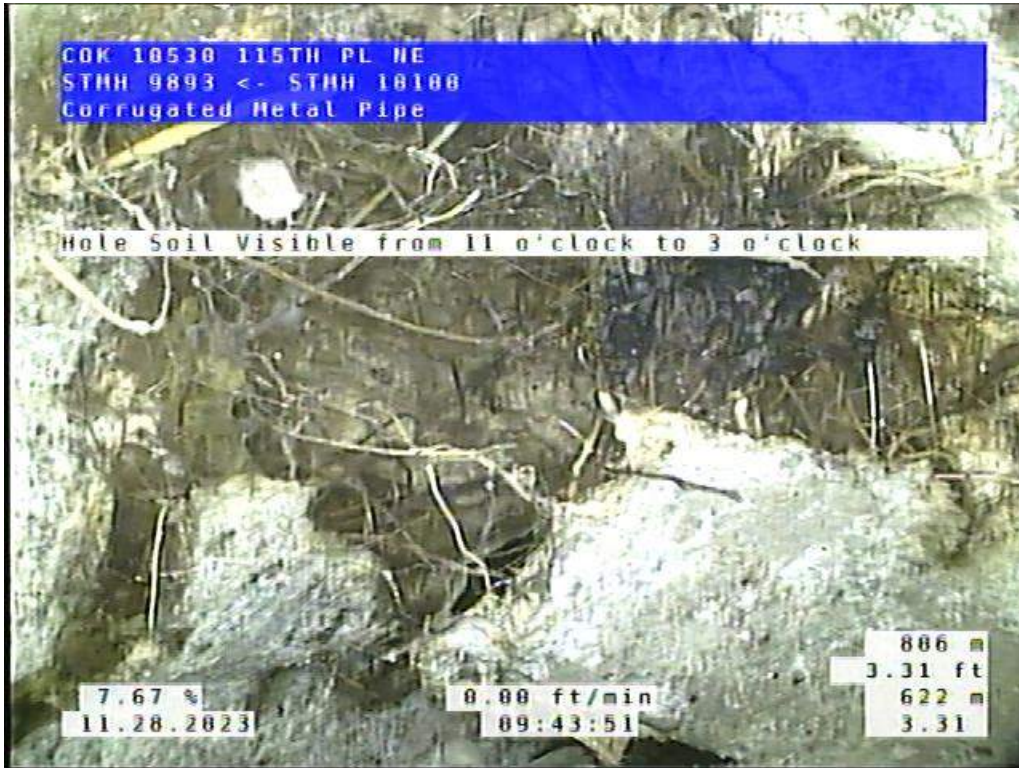
Site 1, Photo #3: 3.31 ft upstream of #10100
