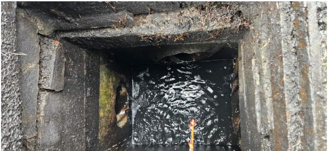
Site 5, CB#11247 –Type 1 catch basin (direction north at top image)
