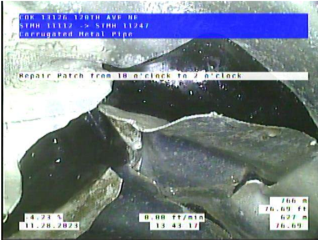
Site 5, Photo #5: 76.69 ft downstream of #11112
