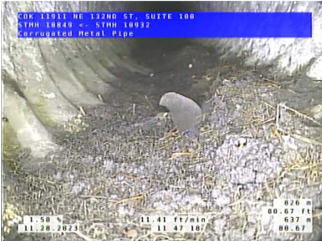
Site 3, Photo #2: 80.76 ft downstream of #10932
