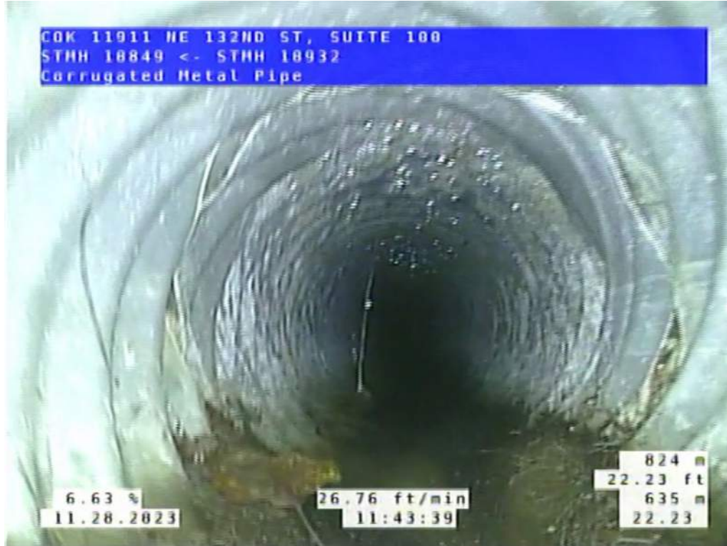
Site 3, Photo #1: 22.23 ft downstream of #10932
