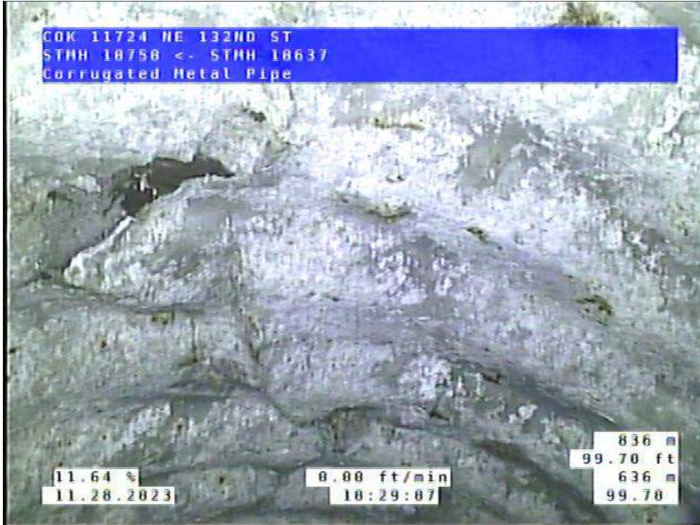
Site 2, Photo #7: 99.78 ft upstream of #10637
