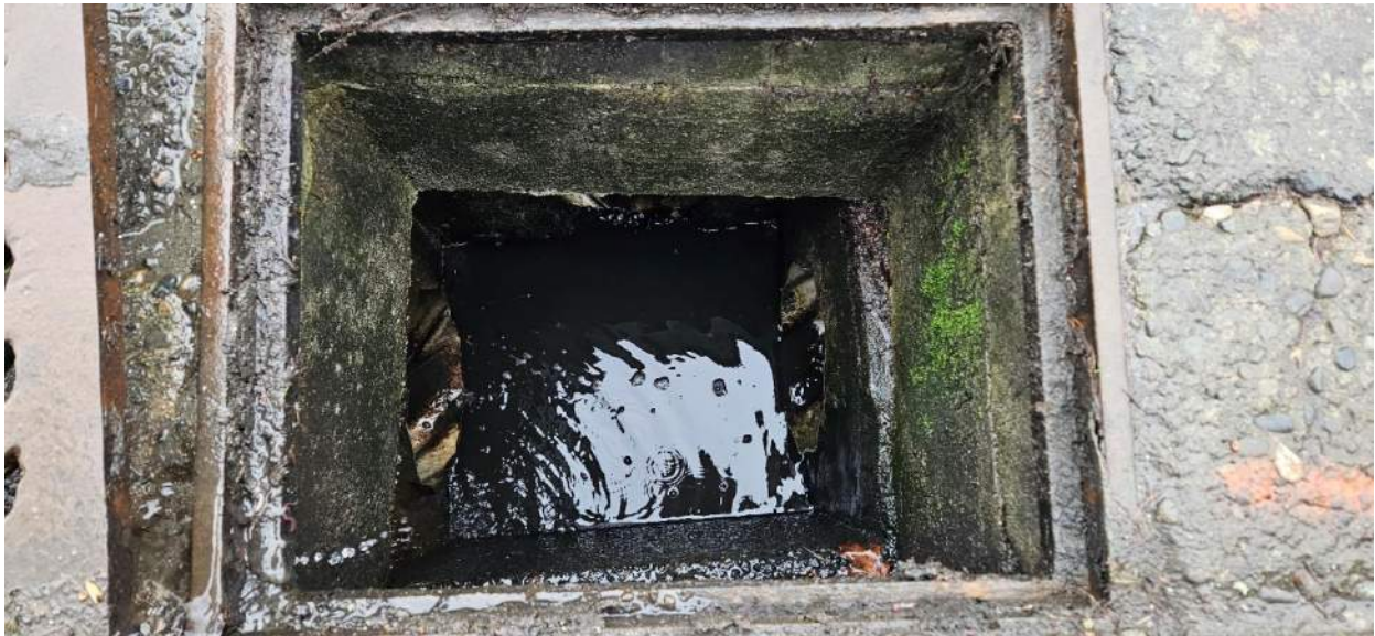
Site 4 and 5, CB#11112 –Type 1 catch basin (direction north at top image)
