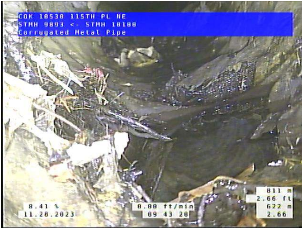
Site 1, Photo #1: 2.66 ft upstream of #10100
