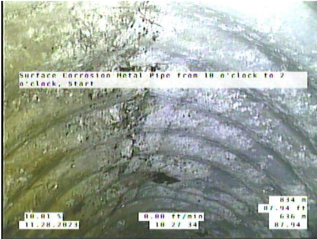
Site 2, Photo #6: 87.94 ft upstream of #10637
