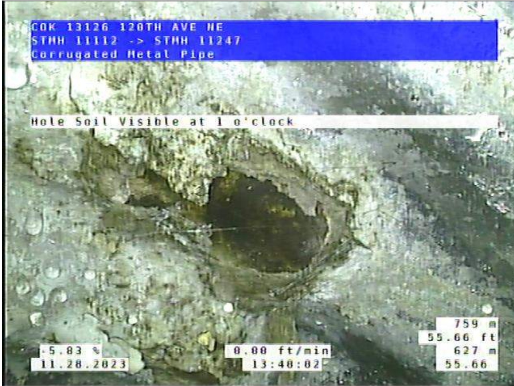
Site 5, Photo #2: 55.66 ft downstream of #11112
