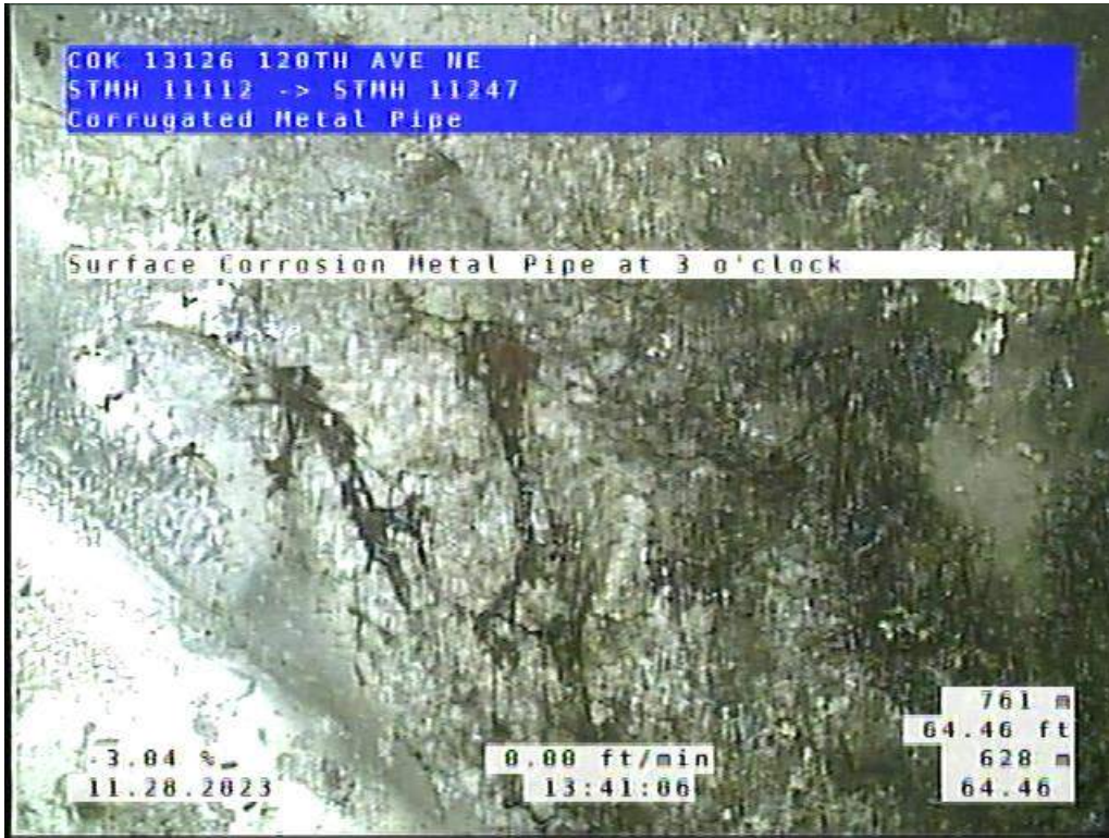
Site 5, Photo #3: 64.46 ft downstream of #11112
