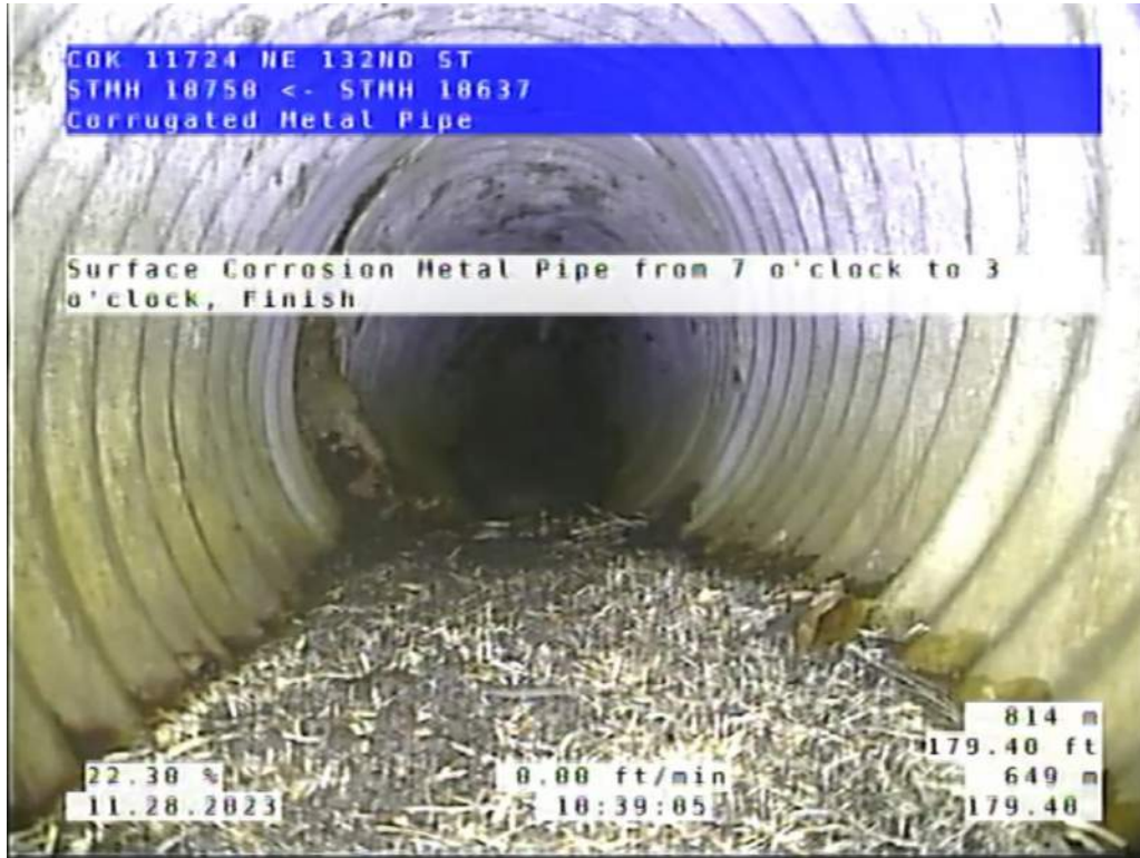
Site 2, Photo #8: 179.40 ft upstream of #10637
