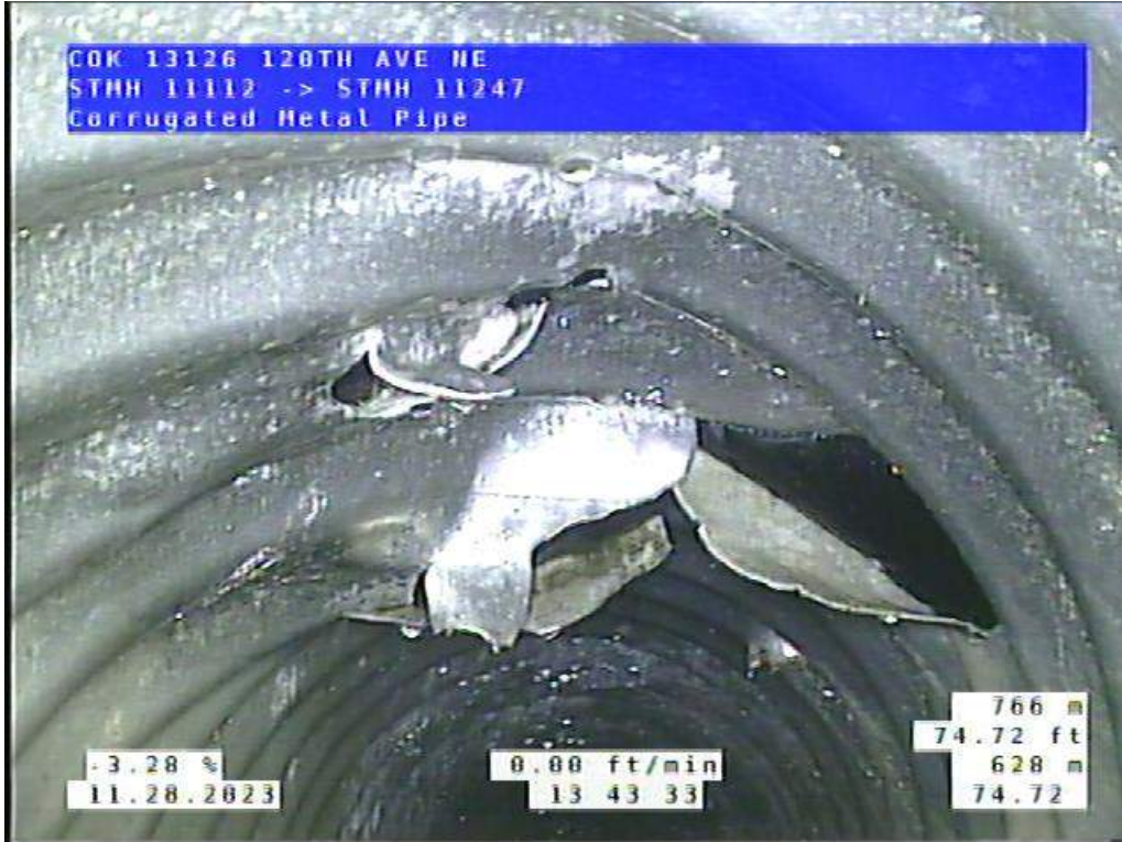
Site 5, Photo #4: 74.72 ft downstream of #11112
