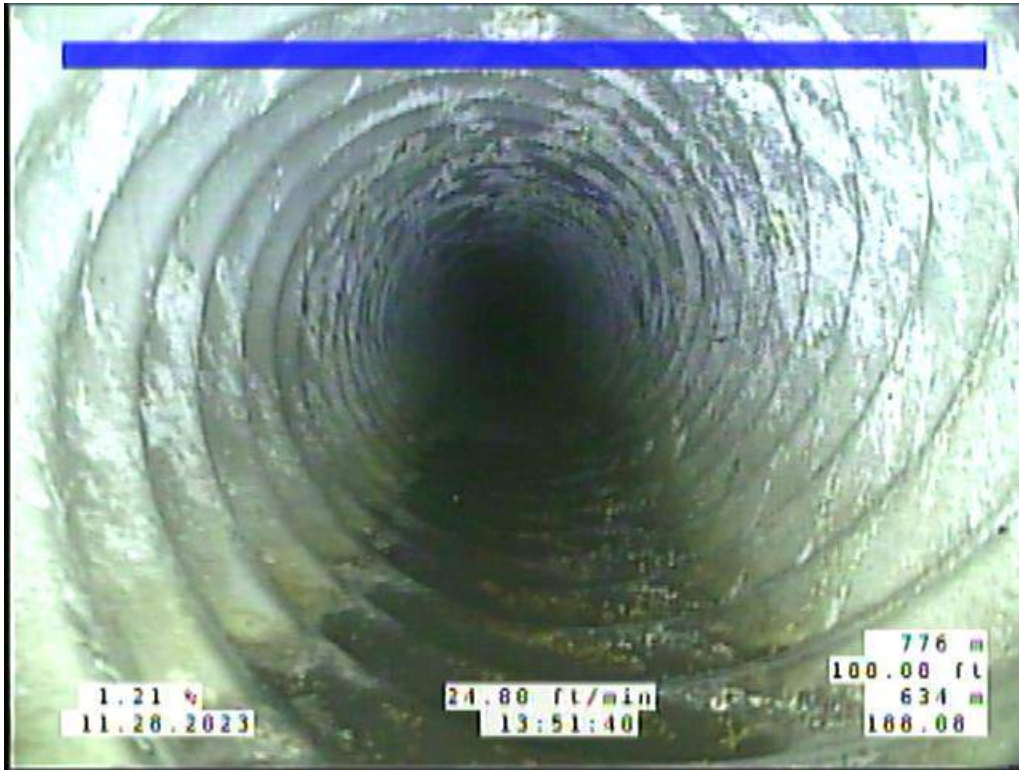
Site 5, Photo #7: 188.08 ft downstream of #11112
