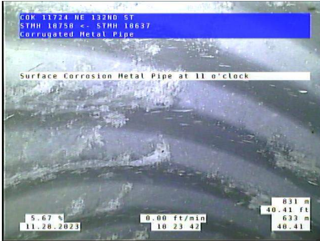
Site 2, Photo #4: 48.41 ft upstream of #10637
