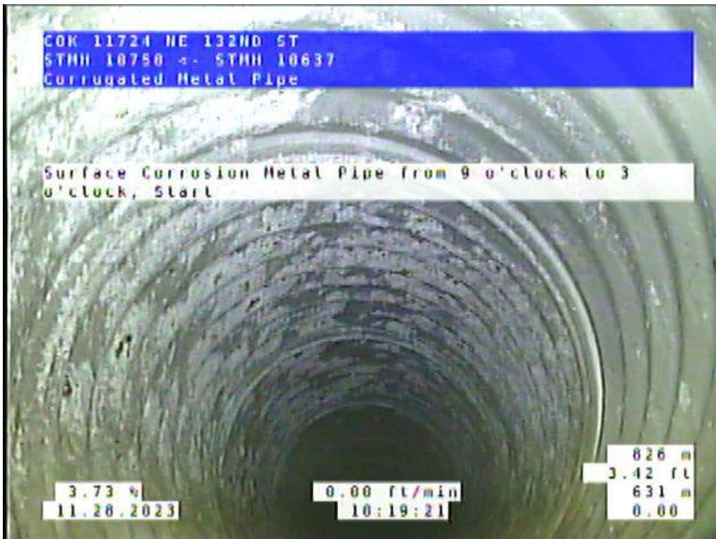
Site 2, Photo #1: 0.00 ft upstream of #10637
