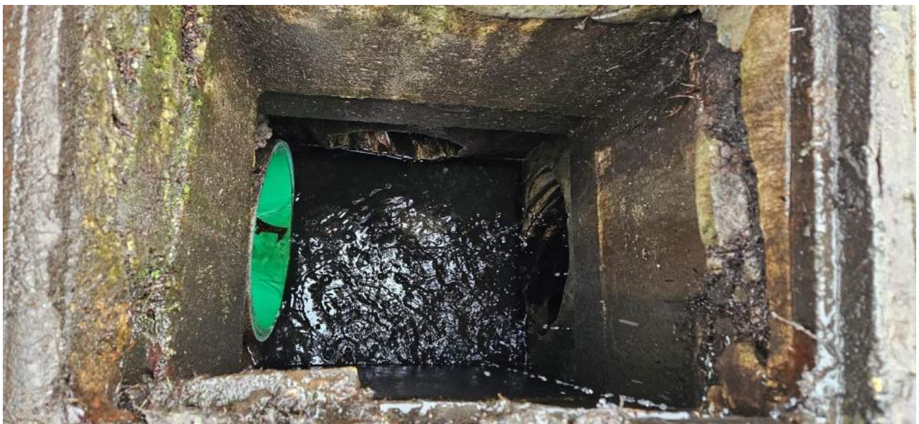
Site 2, CB#10637 –Type 1 catch basin (direction north at top image)
