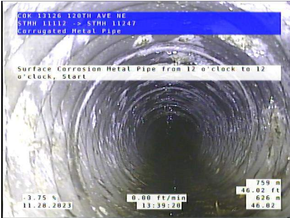
Site 5, Photo #1: 46.02 ft downstream of #11112
