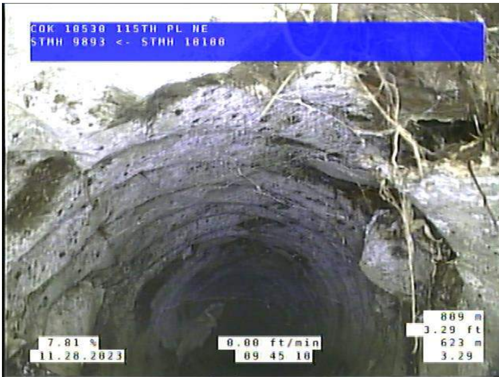
Site 1, Photo #2: 3.29 ft upstream of #10100
