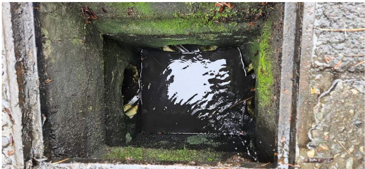
Site 3 and 4, CB#10932 –Type 1 catch basin (direction north at top image)
