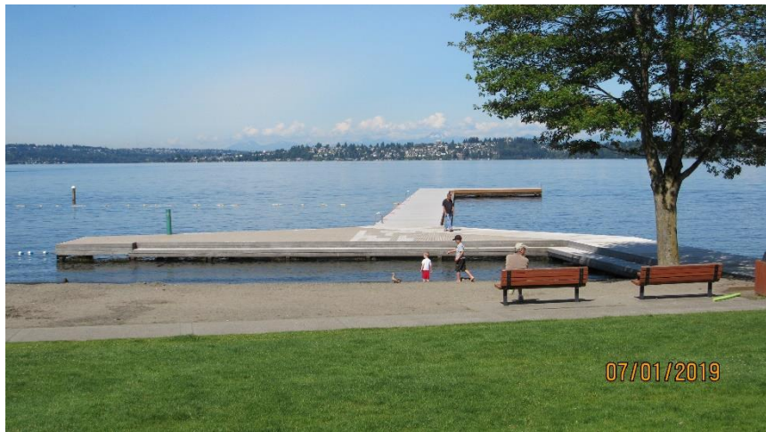
Photo 20. Pier (8), Looking West, Houghton Beach Park.
