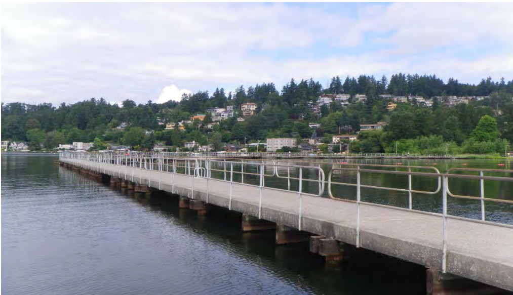
PHOTO No. 1: Juanita Beach Park, Looking West - The structure is built on treated piles with double cap timbers at each bent. Inspection noted that the piles have been notched on both sides to provide a ledger for the cap timbers. The structure has a concrete deck system, as well as an old deteriorated timber wave baffle system and diagonal steel tension rods located in areas underwater and in the plane of the deck.
