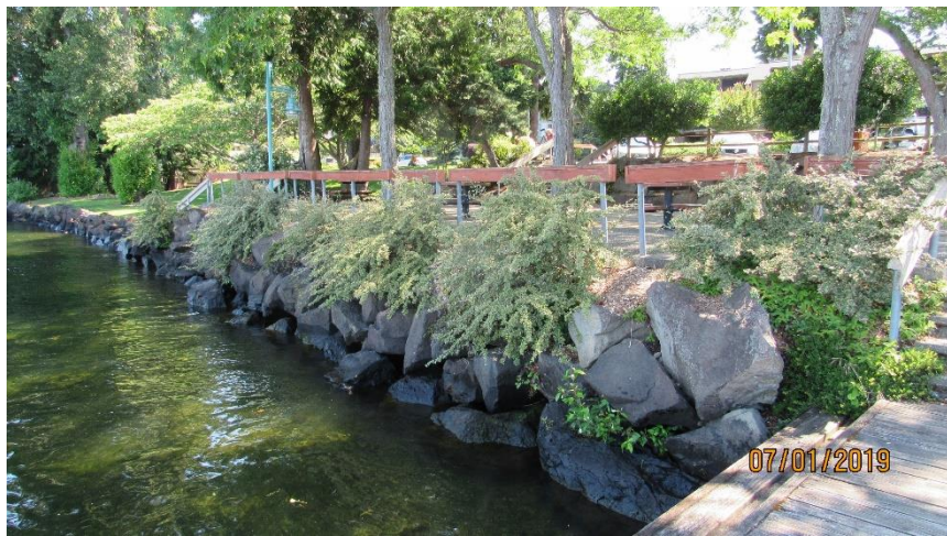
Photo 34. Riprap Bulkhead (5), Marsh Park.
