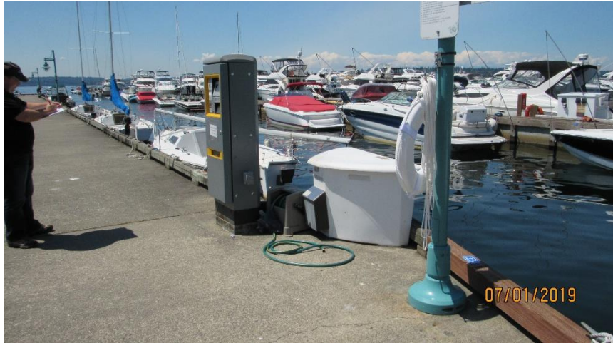
Photo 47. Pay Kiosk and Light Fixture on Pier (1), 2 nd Ave. South Dock.
