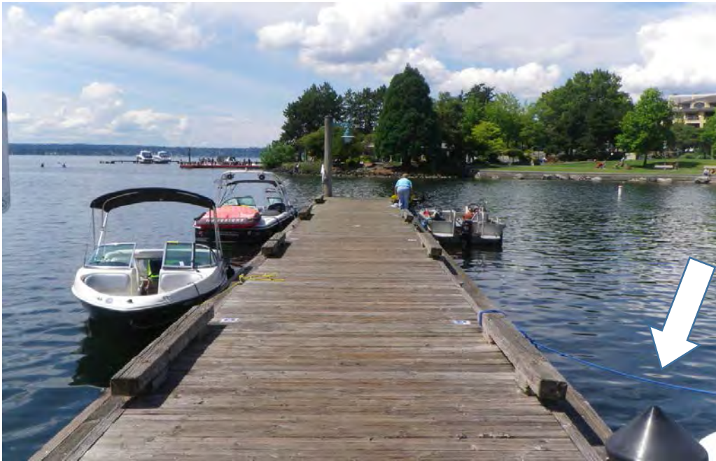
PHOTO No. 3: Eastern Finger, Looking North - Note the generally good condition of the timber decking and the arrow indicating a plastic pile cap located on the Bent 5, Row A Pile.
