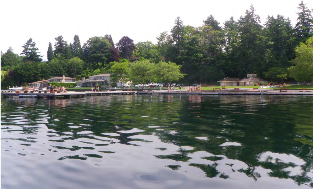
PHOTO No. 1: Waverly Park Pier, Looking Northeast - The pier is constructed on timber piling with timber caps, stringers and decking.
