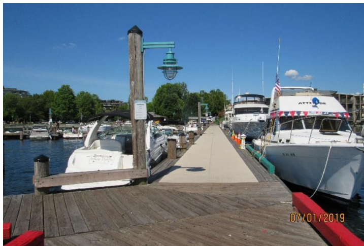
Photo 78. Light Poles on Pier (8), Marina Park.
