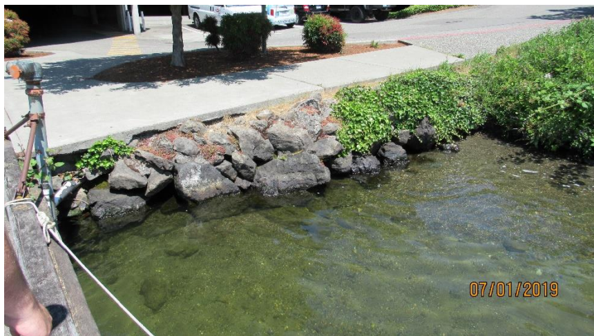
Photo 45. Riprap Bulkhead (1) Looking East, 2 nd Ave. South Dock.
