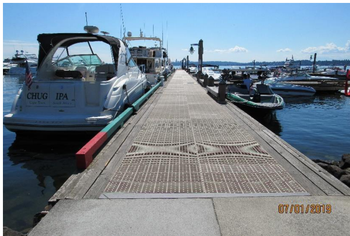
Photo 66. Pier (8) Entrance Looking Southwest, Marina Park.
