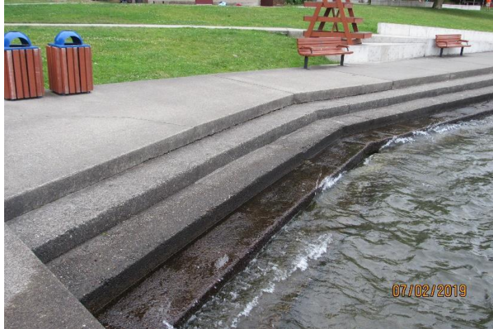
Photo 82. Concrete Steps & Sidewalk (4) Looking South, Waverly Park.
