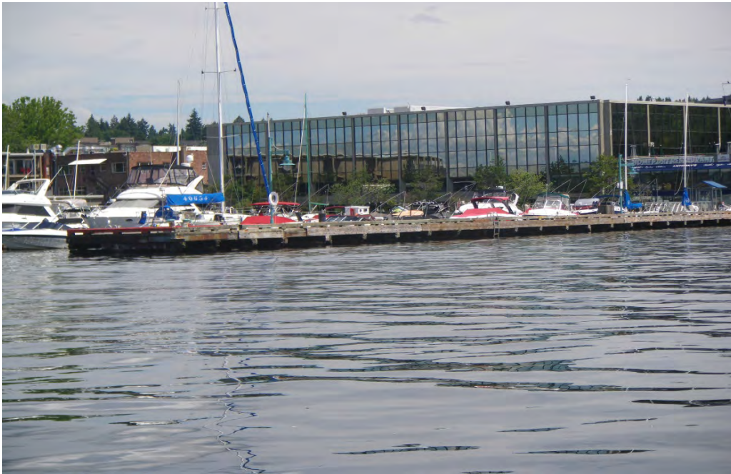
PHOTO No. 1: Second Avenue South Pier, Looking Northeast - The structure is constructed on timber piles with treated caps and stringers, supporting a galvanized sub pan and poured in-place concrete deck. Note that pleasure craft moored along the north side of the pier.
