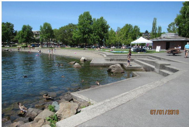
Photo 52. Conc. Steps & Sidewalk (3) and Beach (4) Looking North, Marina Park.
