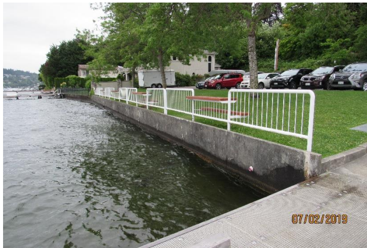
Photo 84. Ecology Block Bulkhead (5) Looking North, Waverly Park.
