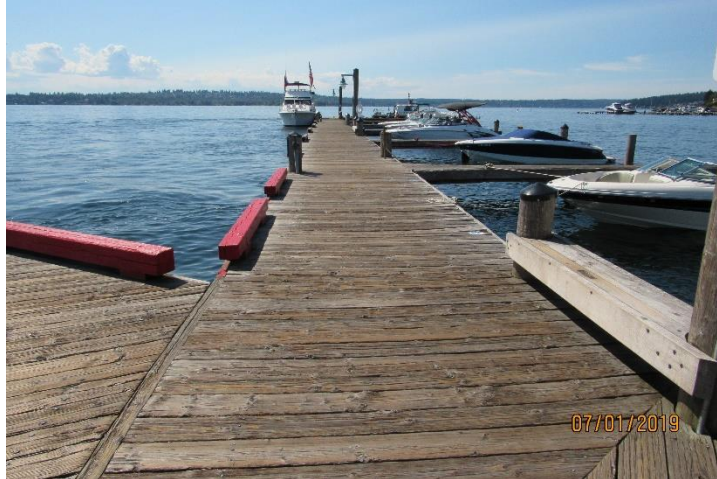
Photo 77. Benches and Bull Rails on Pier (8), Marina Park.
