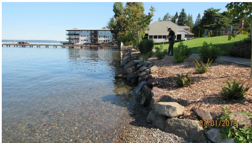
Photo 15. Concrete Revetment (8) Looking North, Houghton Beach Park.
