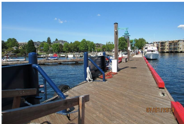
Photo 67. Pier (8) Superstructure, Marina Park.
