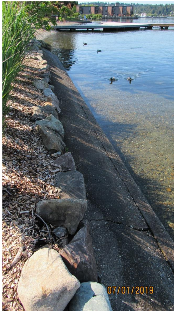
Photo 17. Concrete Revetment (8) Looking South, Houghton Beach Park.
