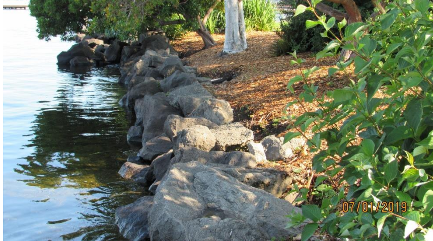
Photo 4. Riprap Bank Slope (3) Looking North, Houghton Beach Park.
