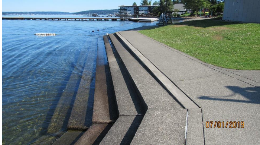
Photo 10. Curved Concrete Steps and Sidewalk (5), Houghton Beach Park.
