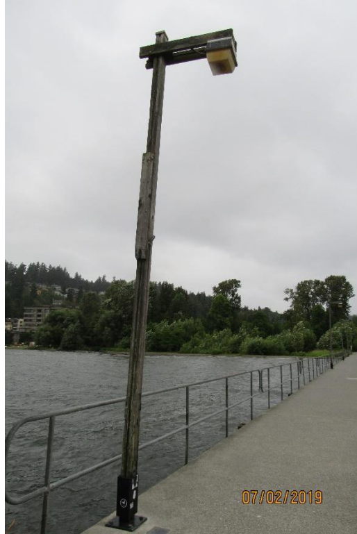
Photo 93. Light Pole on Pier (1), Juanita Beach Park.
