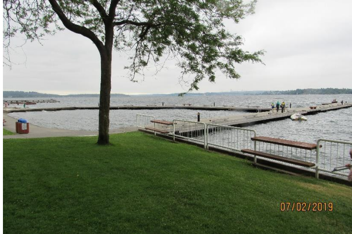
Photo 85. Ecology Block Bulkhead (5) and Pier (6) Looking Southwest, Waverly Park.
