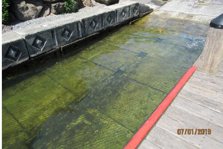
Photo 65. Conc. Boat Ramp Panels (7), Marina Park.
