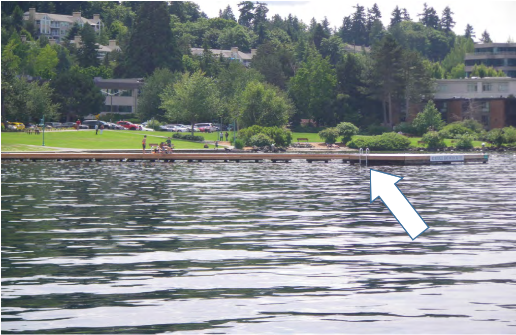
PHOTO No. 1: Houghton Beach Pier, Looking Southeast - Note the swim ladder located on the north side of the on the Pierhead. The structure is constructed using timber substructure piles, caps and stringers with a plastic grate decking.
