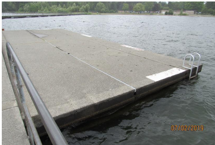
Photo 93. Concrete Swim Float on Pier (1), Juanita Beach Park.
