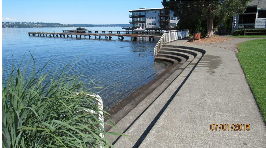
Photo 18. Concrete Steps and Sidewalk (8) Looking North, Houghton Beach Park.
