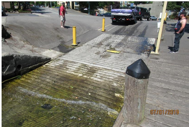
Photo 64. Conc. Boat Ramp (7), Marina Park.
