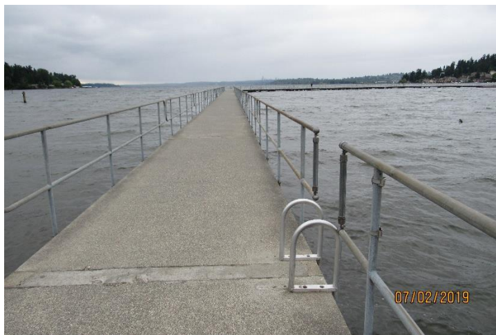
Photo 90. Safety Ladder and Handrails on Pier (1), Juanita Beach Park.
