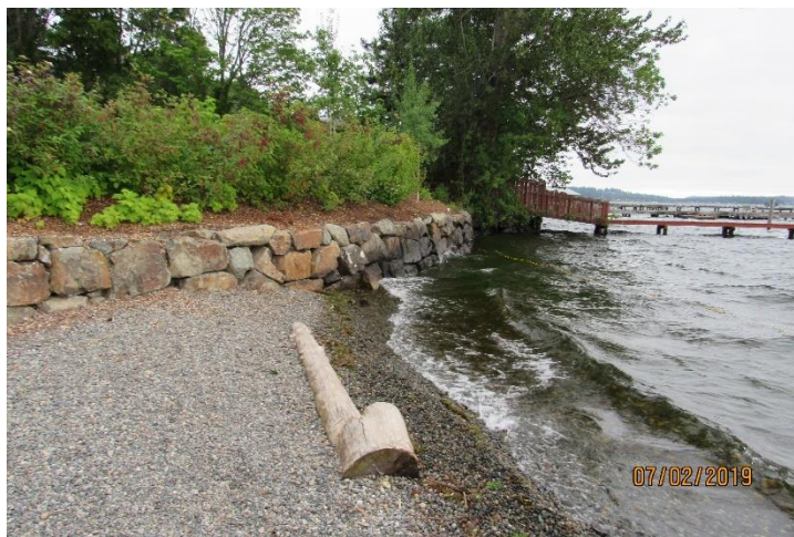
Photo 79. Riprap Bulkhead (1) and Beach (2) Looking South, Waverly Park.
