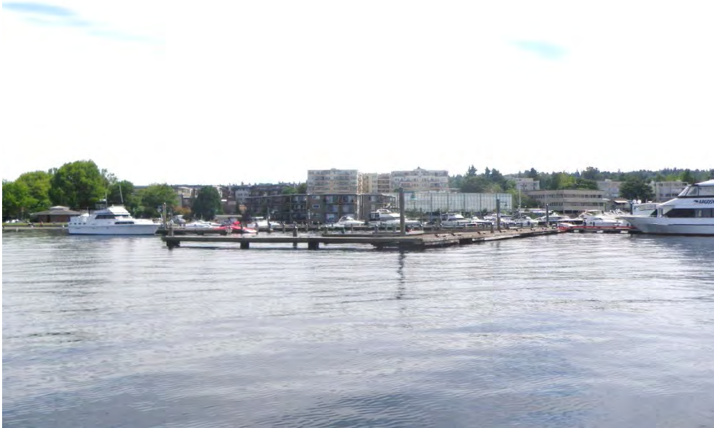
PHOTO No. 1: Marina Park, Main Pier, Looking Southeast - The structure is constructed using typical timber construction with treated timber piles, pile caps, stringers, and decking. Note that a number of the piles extend above the elevation of the deck.
