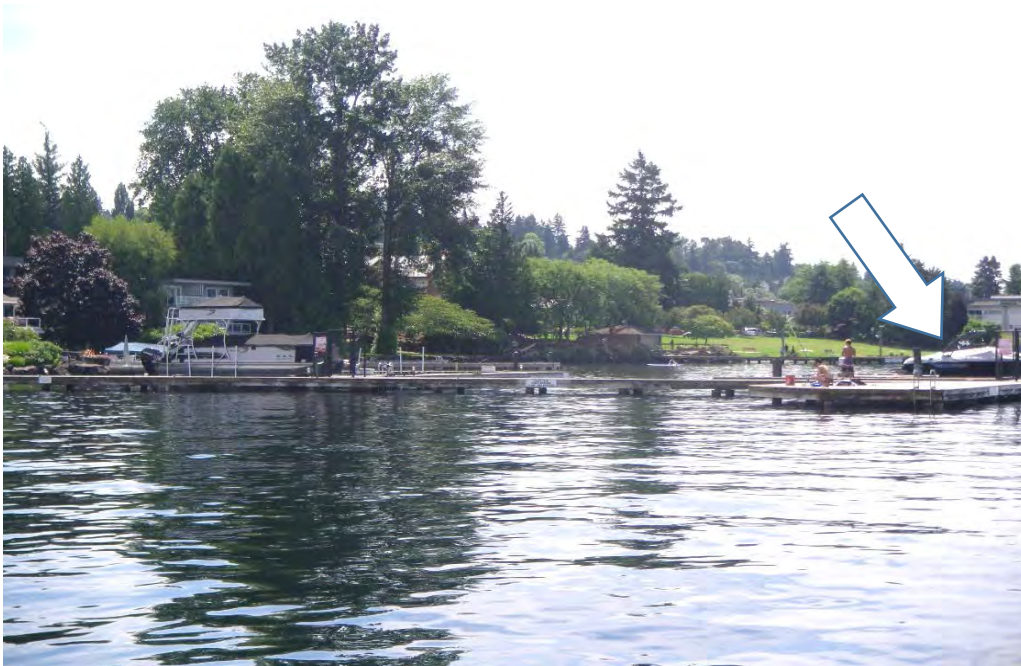
PHOTO No. 1: Settler's Landing Pier, Looking Southeast - The pier is constructed with treated timber piles, and superstructure, including pile caps, stringers, and decking. Note the boat moored to one of two privately owned moorage piers that extend to the south and were not included in the investigation.
