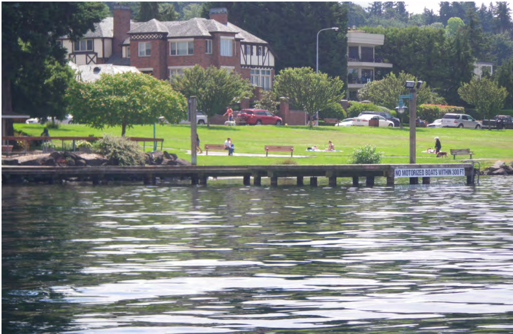
PHOTO No. 1: Marsh Park Pier, Looking Southeast - The structure is supported by treated timber piles and treated superstructure members. Note the two piles which extend above the deck. These are driven piles which act as a light post and sign post.
