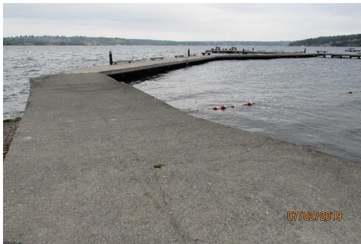
Photo 81. Concrete Pier (3) Looking West, Waverly Park.
