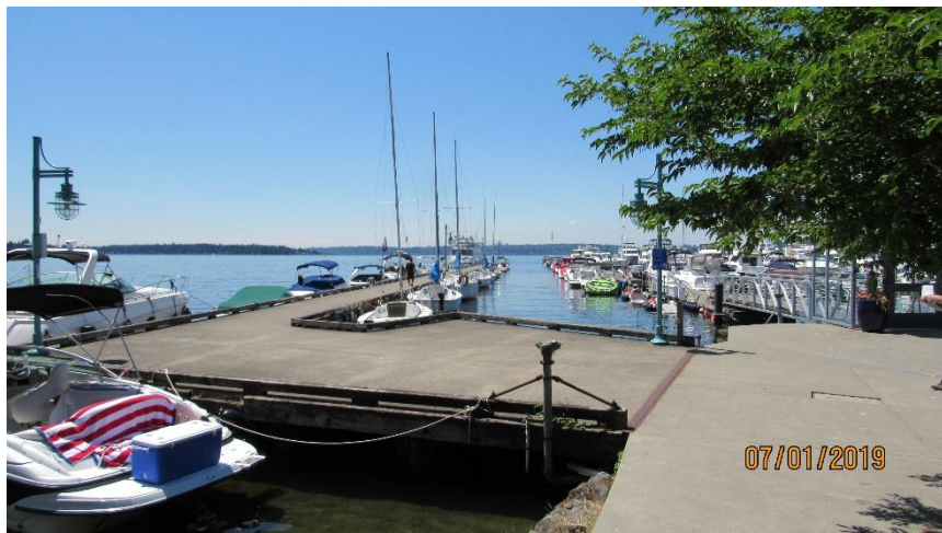
Photo 44. Pier (1) Looking West, 2 nd Ave. South Dock.
