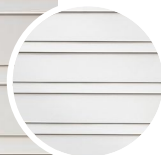
HORIZONTAL LAP SIDING ON EXTERIOR WALLS
