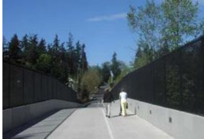
100th Street Pedestrian Bridge over I-405
