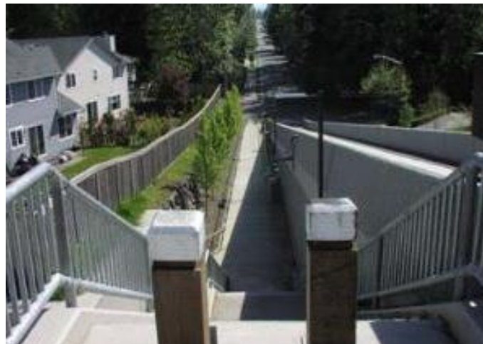
NE 100th Street Emergency/ Nonmotorized-Nonvehicular Overpass
