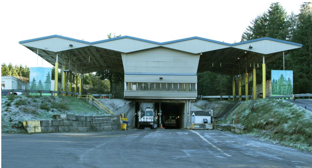
King County Transfer Station
