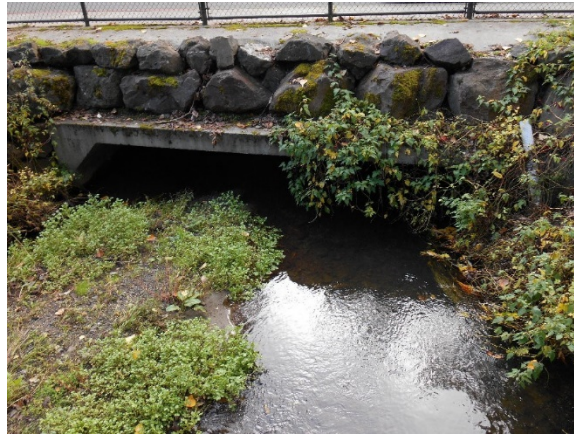
Juanita Creek Fish Passage
