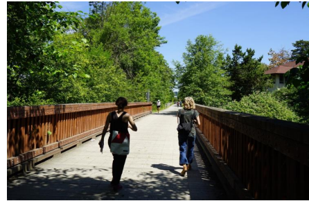
CKC Bridge over 68th Street
