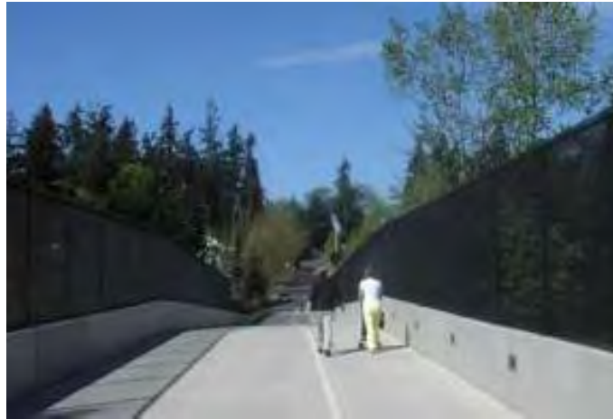
100th Street Pedestrian Bridge over I-405
