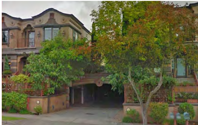
Office Development on Market Street
