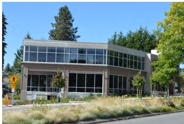
Dibble Office Building
