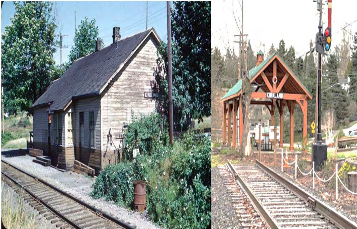
Old train station and new Rotary Central Station picnic pavilion
