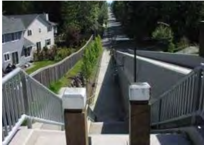
NE 100th Street Emergency/ Nonmotorized Nonvehicular Overpass
