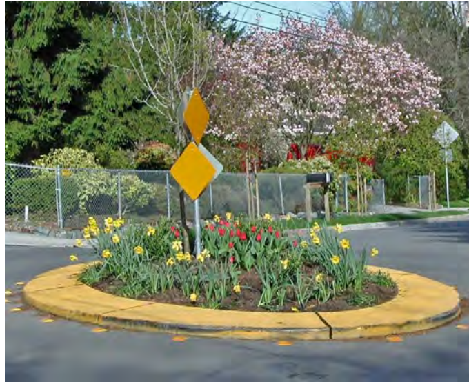
Example of traffic circle installed for slowing down vehicle speed
