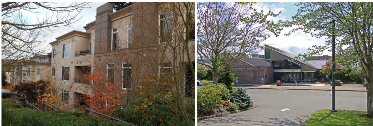
Condominiums on 4th Avenue and 2nd Street and Kirkland City Hall at 123 5th Avenue
