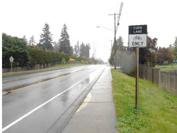
Bike lane along 132nd Ave NE
