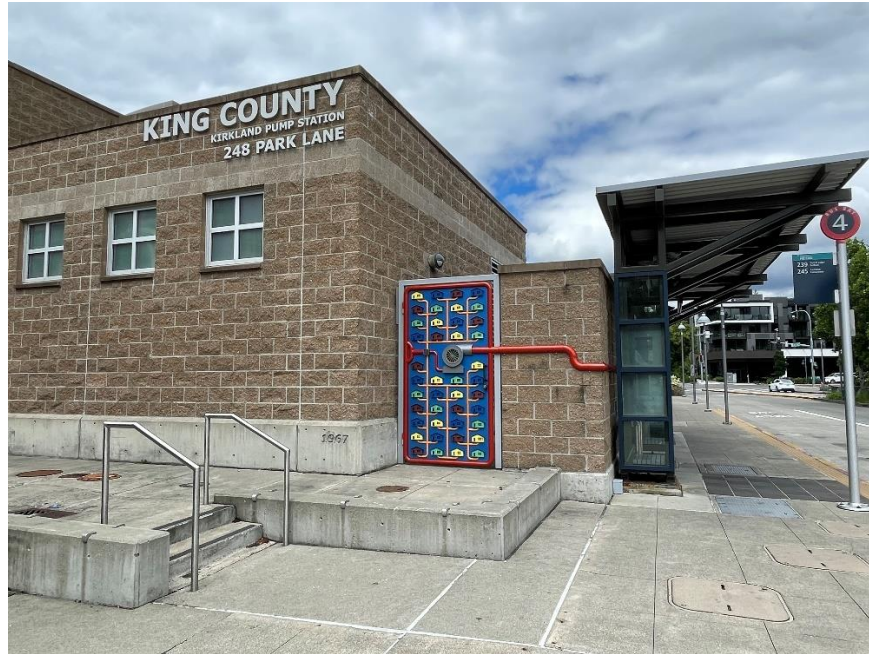
King County pump station in downtown Kirkland
