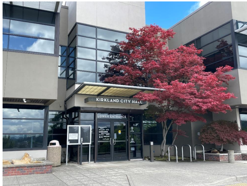
Kirkland City Hall, Lower entrance
