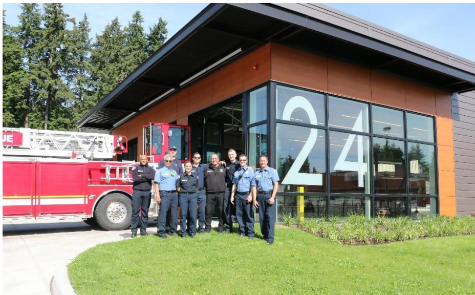
Fire Fighters at Station 24
