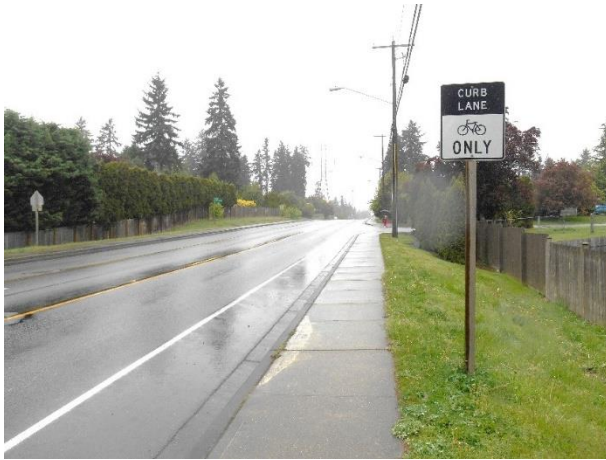
Bike lane along 132nd Ave NE
