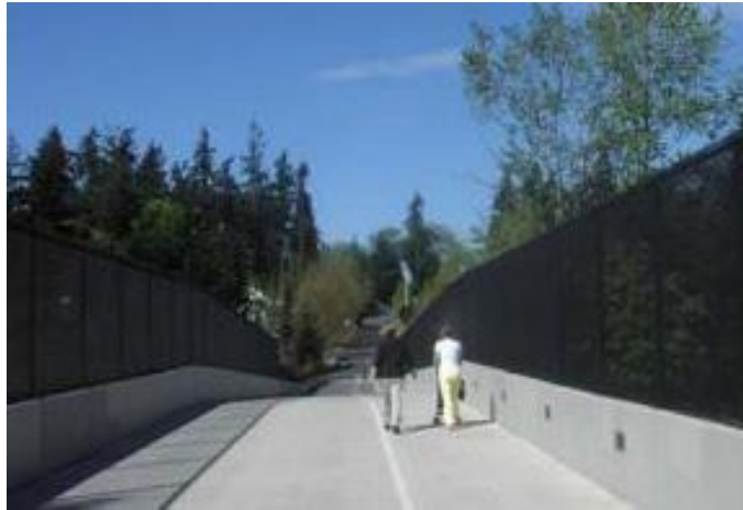
100th Street Pedestrian Bridge over I-405
