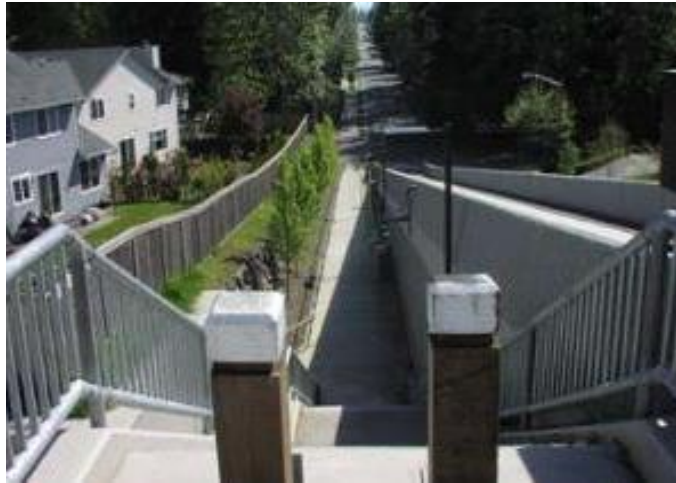
NE 100th Street Emergency/ Nonmotorized Nonvehicular Overpass
