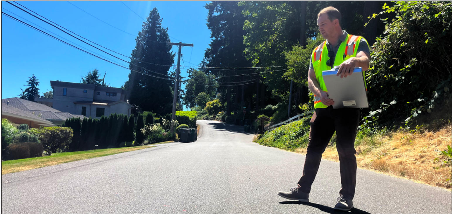
Will Denton, Kirkland's streets engineer, inspects Finn Hill's Northeast 110th Place, near Juanita Drive, to ensure it is in good enough condition for street sealing. Kirkland's contractor in August will slurry seal more than 30 sections of neighborhood roads in Finn Hill and Juanita.
