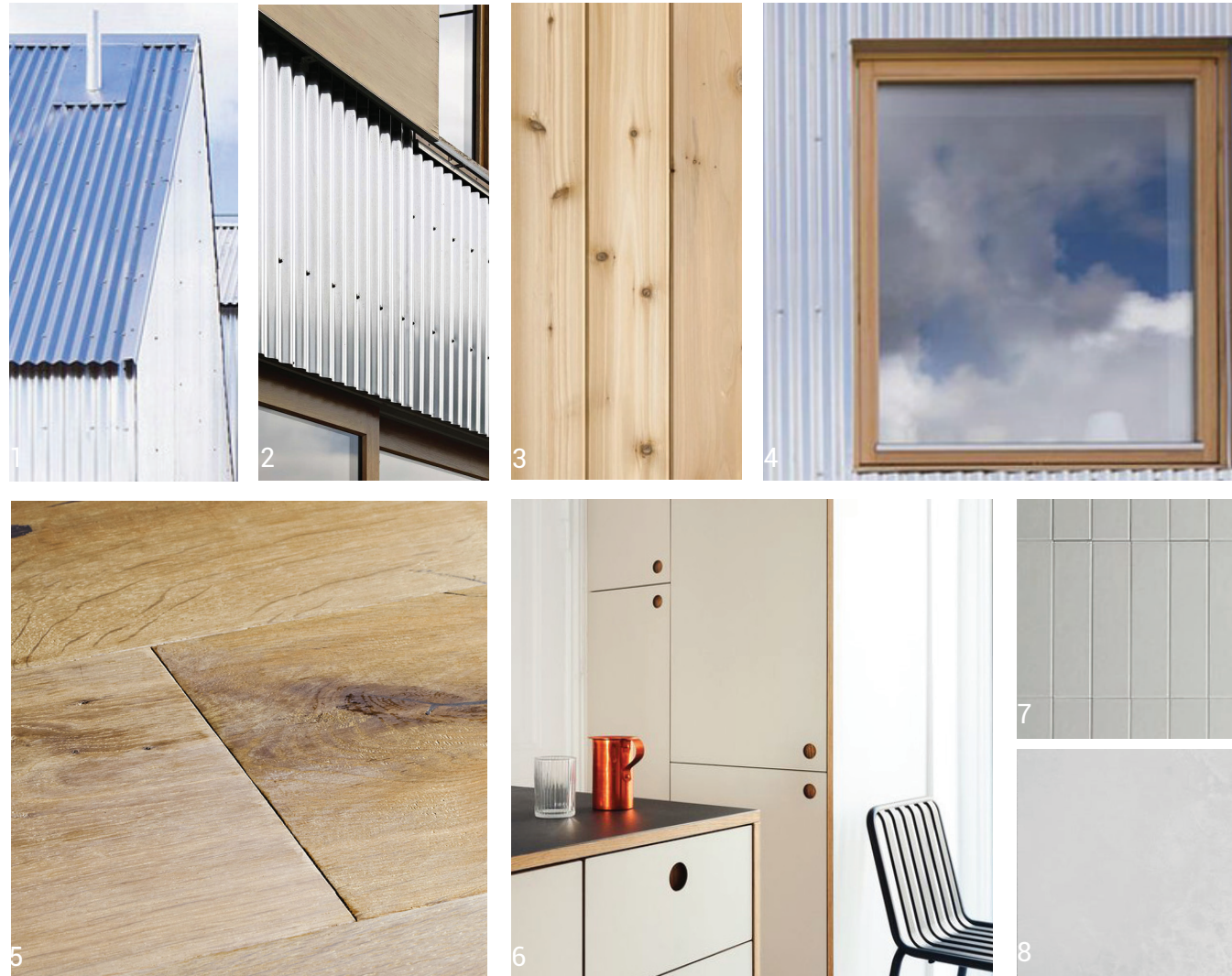
MATERIALS: 1. Corrugated Metal Roofing. 2. Corrugated Metal 3. Alaskan Cedar Hardwood decking 4. Wood window 5. White oak floor, soap treated. 6. Plywood cabinets and paperstone countertop 7. Vertical ceramic tiles 8. Light grey microcement.
