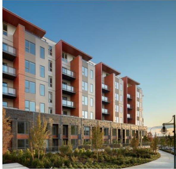
Figure 17: District Context on 6th Street
