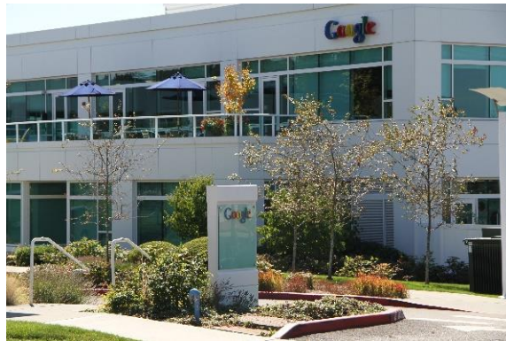
Figure ED-1: Google offices in Kirkland
