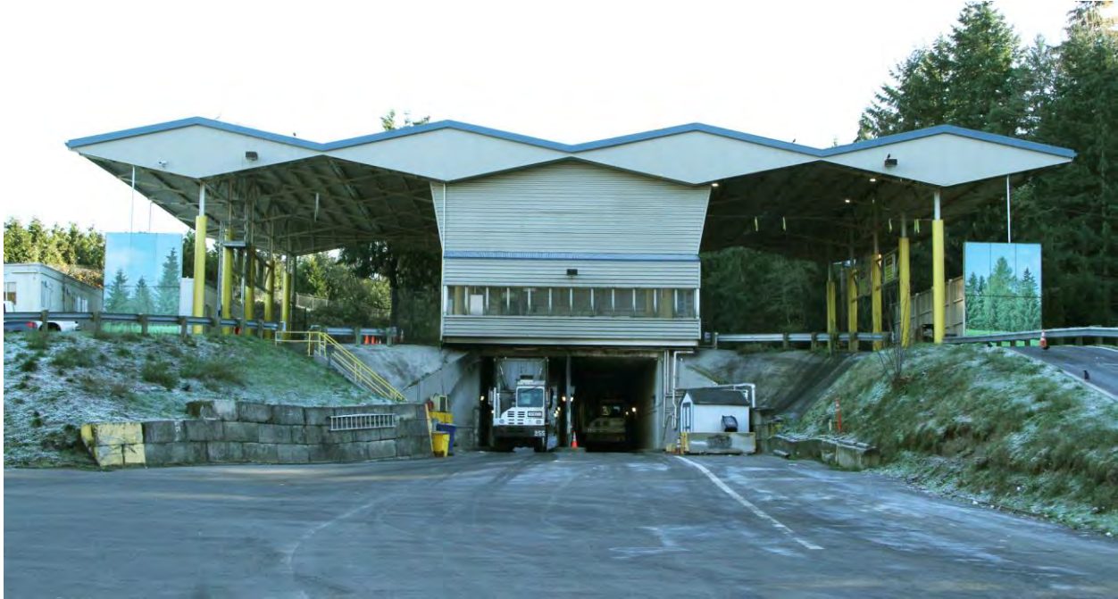
King County Transfer Station
