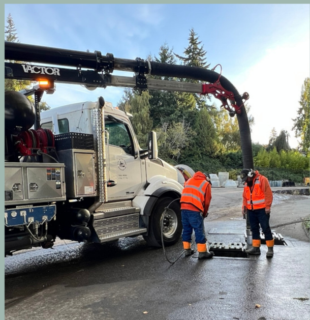
Above: Crews performing maintenance on a structure with City vactor truck.
