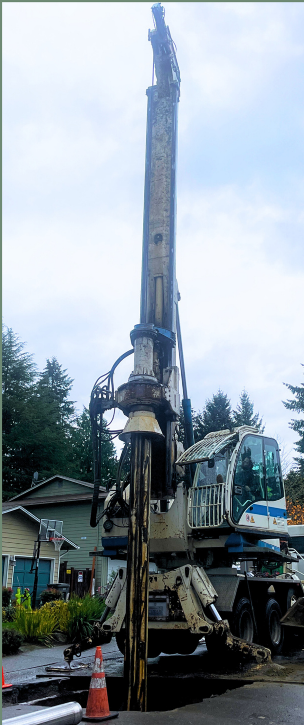
Above: Construction of infiltration facility in residential area.
