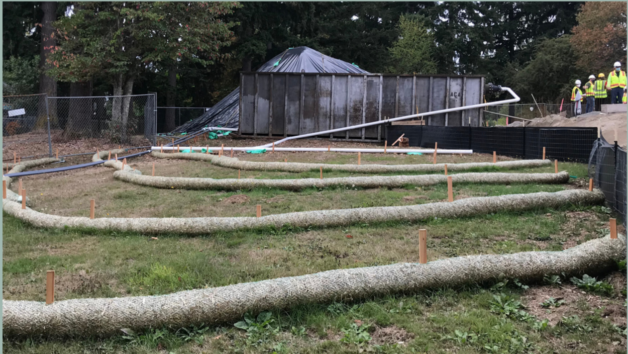
Above: Erosion control at 132nd Square Park, Stormwater Park.
